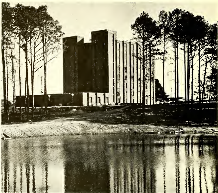
PARKER HALL . . . Residence For Men
