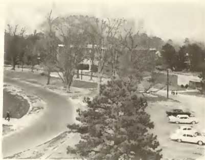
AERIAL VIEW OF CHOWAN
