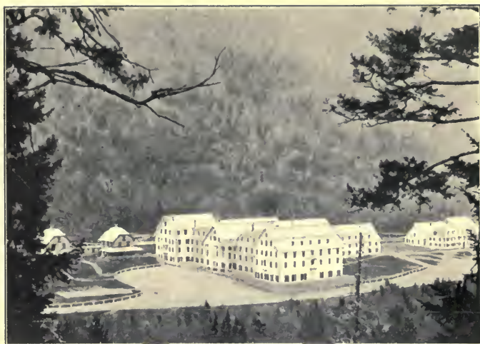
THE OLD PROFILE HOUSE, OPENED 1853, CLOSED 1905
