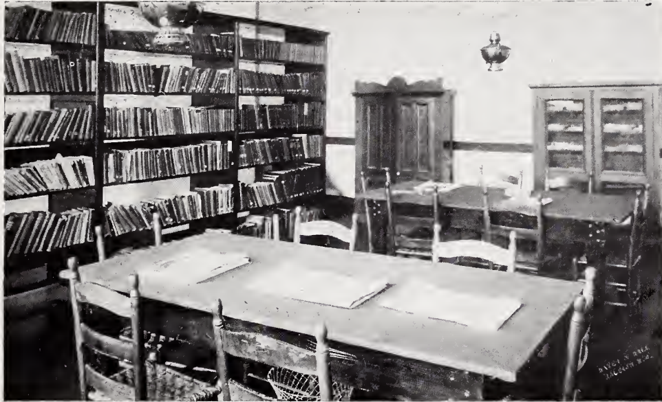
LIBRARY AND READING ROOM
