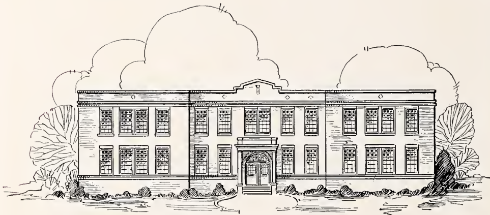
NEW VOCATIONAL BUILDING
