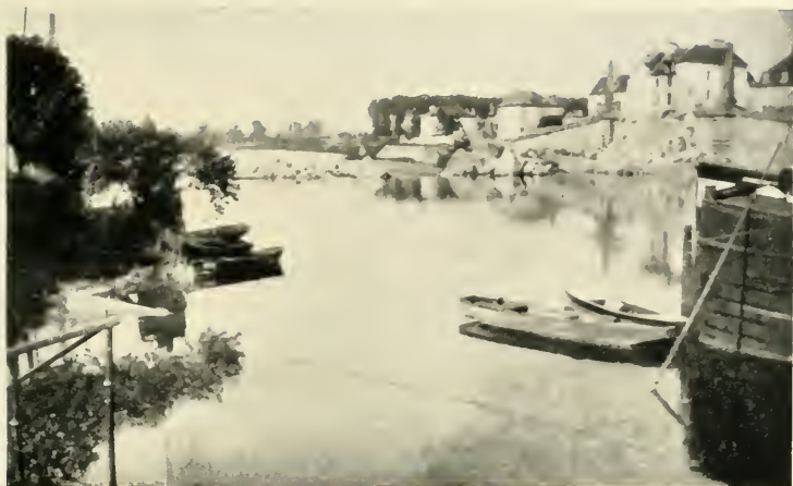
BRIDGE OVER THE OISE DESTROYED DURING THE RETIREMENT.
