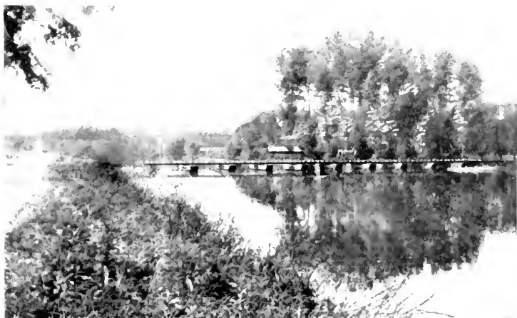
PONTOON BRIDGE OVER THE AISNE NEAR ST. MARGUERITE.
