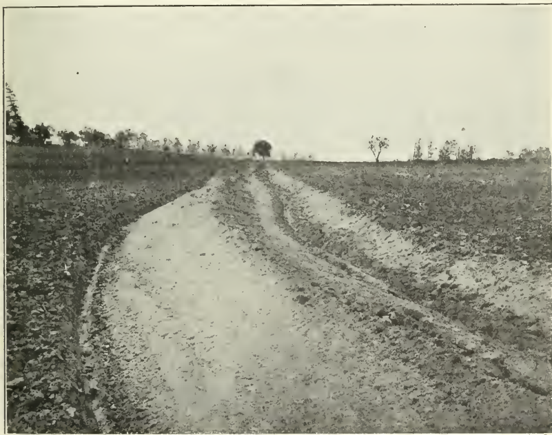
FIG. 4.—Terrace bank thrown up with a road scraper. The sharp depression on the upper side will be eliminated when the area is plowed over, and the water will then spread over a broader surface.
