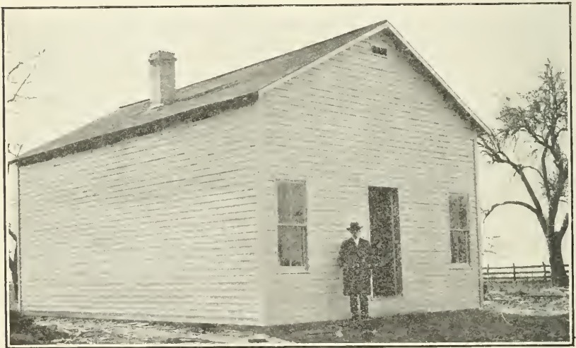
FIG. 1.—Exterior view of a building constructed solely for the good preservation of seed corn. It has a concrete basement and flue. Warm air passes from the basement through openings in the floor, ascends through the corn, and escapes through ventilators.
