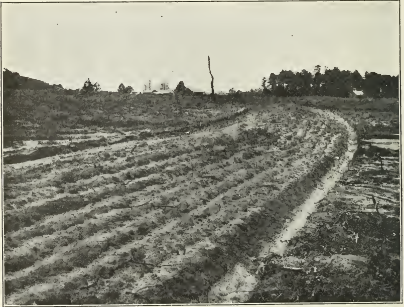
FIG. 3.—The first steps in constructing a Mangum terrace. A backfurfrowing area centers along the grade line.
