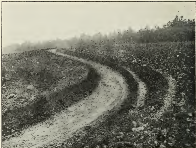
FIG. 5.—The first step in making a terrace with a road scraper when only the upper side is scraped. The lower side will be made the center of the backfurfrowing area, 15 or 20 feet wide.
