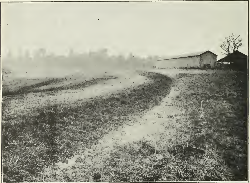
FIG. 9.—The Mangum terrace on steep pasture land. When covered with sod this terrace will last indefinitely with little or no attention.
