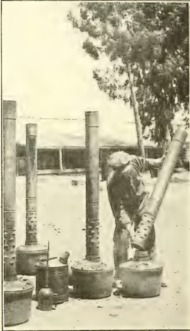
FIG. 93. — The perforated stack gives good combustion but may admit rain-water.
