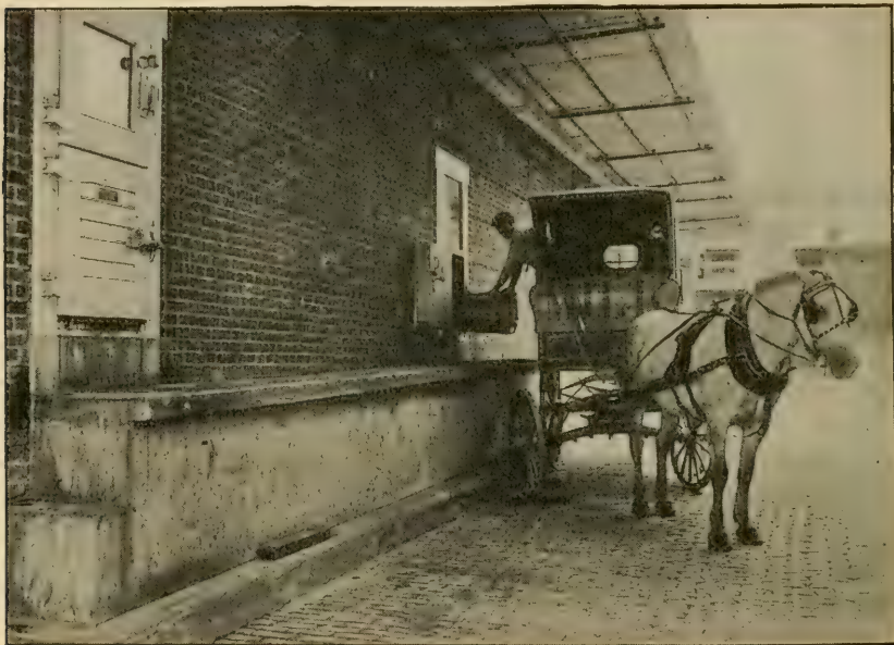
FIG. 6.—Loading delivery wagons at plant using system E . (The second chute was not in use at the time the photograph was taken.) An average of 34.3 wagons per hour were loaded at the three plants using this system. The average time required to load one wagon varied from 1.5 to 2.3 minutes.
