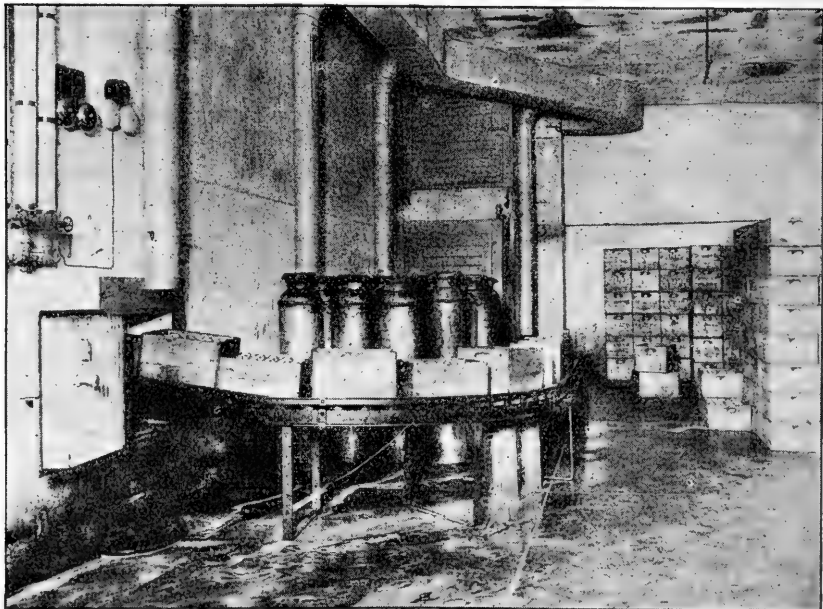
FIG. 14.—Milk-storage room with indirect system of cooling. Note flues through which the cold air is fanned into the room, also system of conveying the milk into the room from the bottling room.
