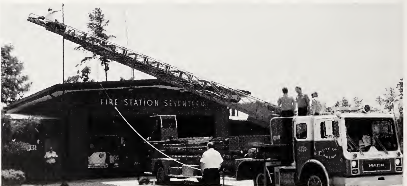
Using Truck 16 to paint flag pole at Station 17 6/93
