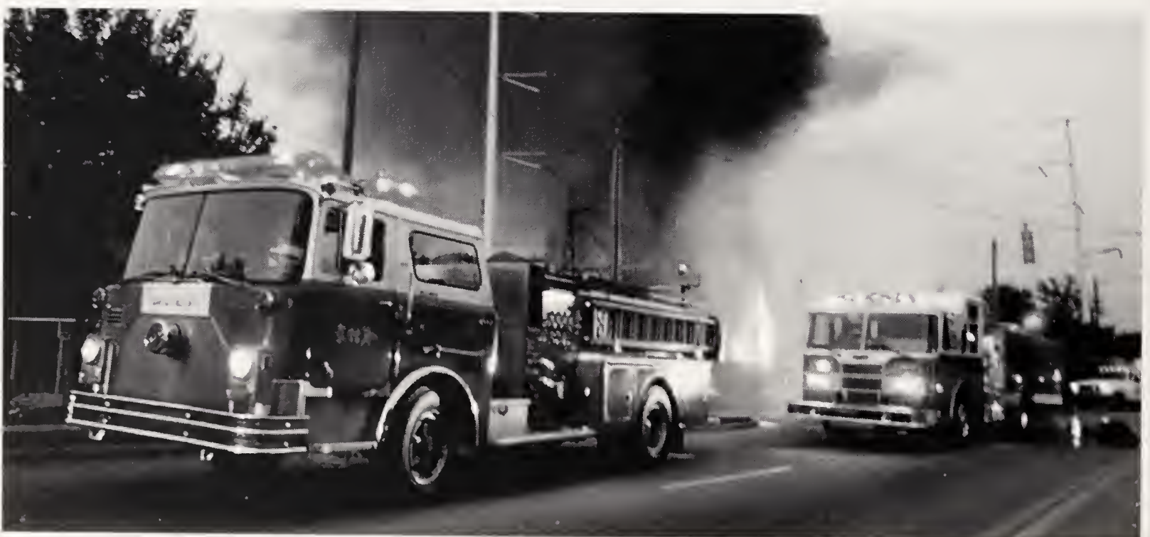
CP&L Substation Fire 7/01
