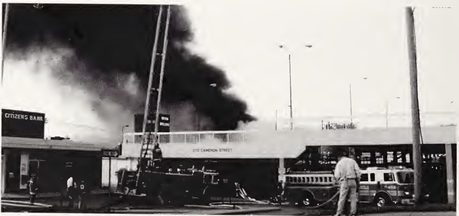
Cameron Village Bryan Building Fire
