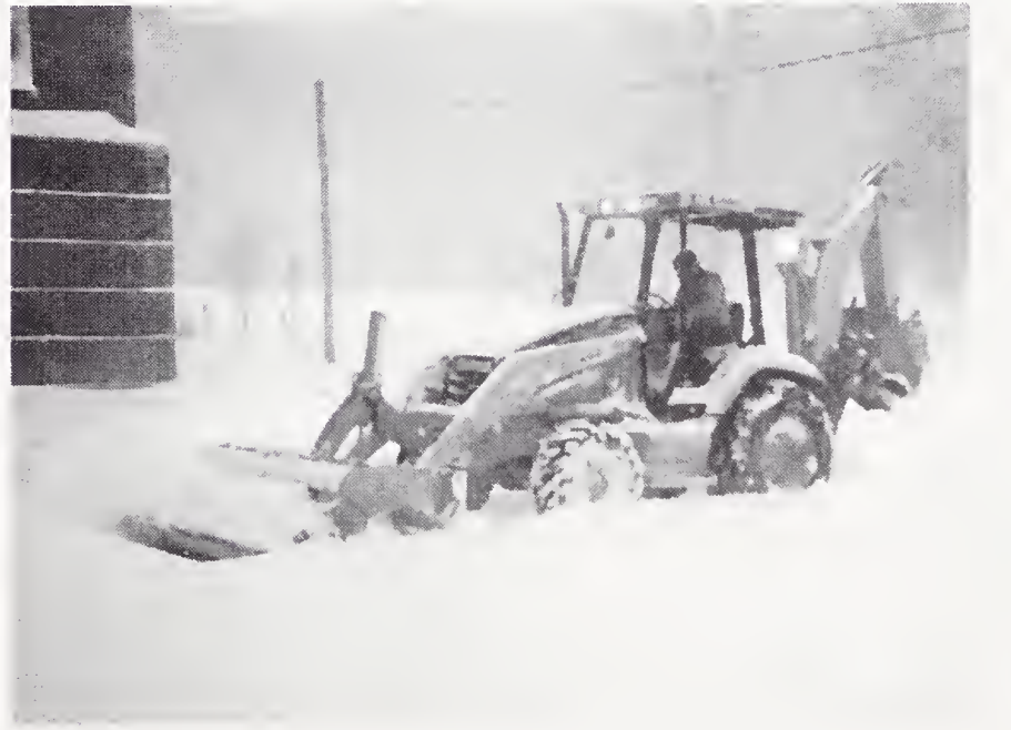
Removing snow from apron at Station 1
