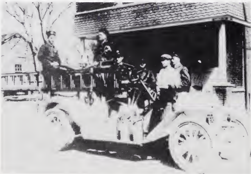
Fire Station Three, E. Hargett Street in 1914
