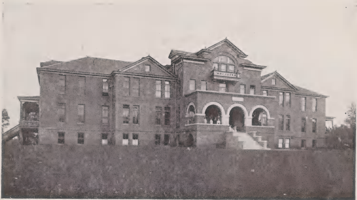
OLD GOODWIN HALL
