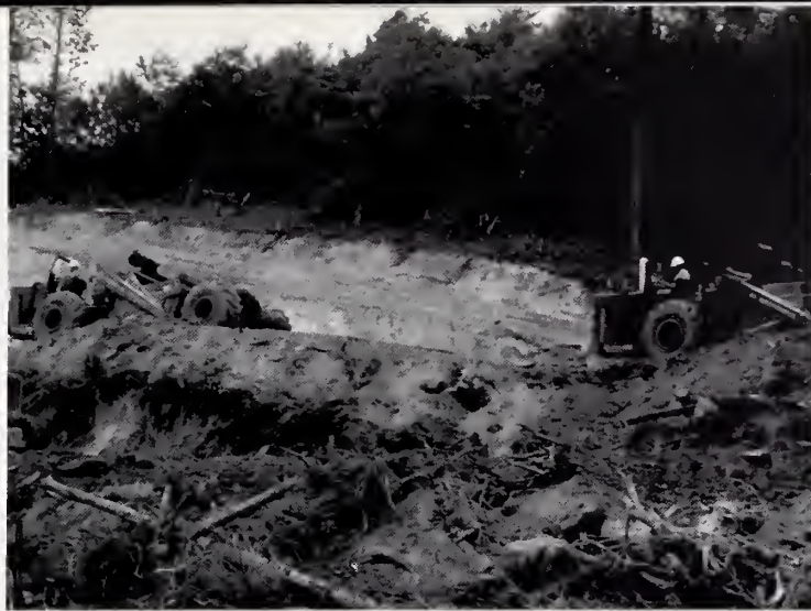
Grading was done early in 1976 for the Technical Arts Building.
