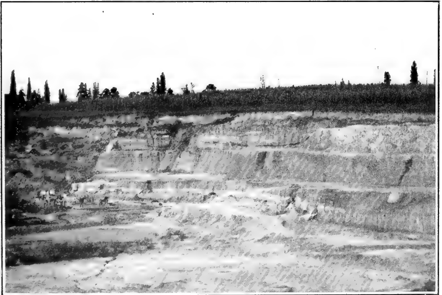
Fig. 2. View in fire-clay pit of National Fireproofing Company, north of Keasbey. The fire clay is dug in pits as at the left. Fireproofing clay overlies the fire clay.
