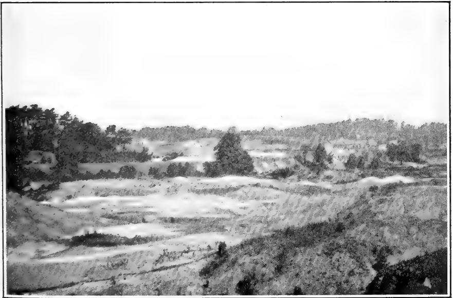
Fig. 2. Two views of the Mutton Hollow opening, Woodbridge, showing the extensive excavations and piles of refuse clay and overburden.
