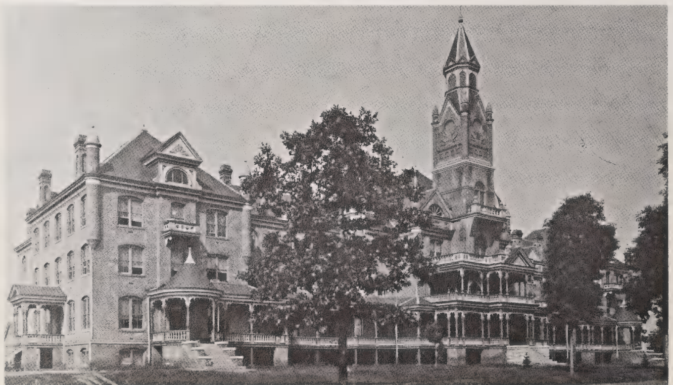
Main Building, as it originally looked before remodeling.
