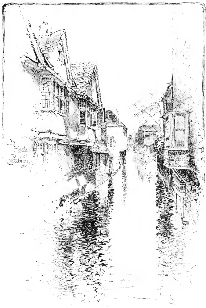
Old Hospital, Canterbury.
