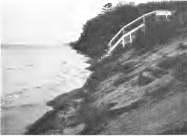
8 May 1973 - View to north; note lack of beach, steep slope.
