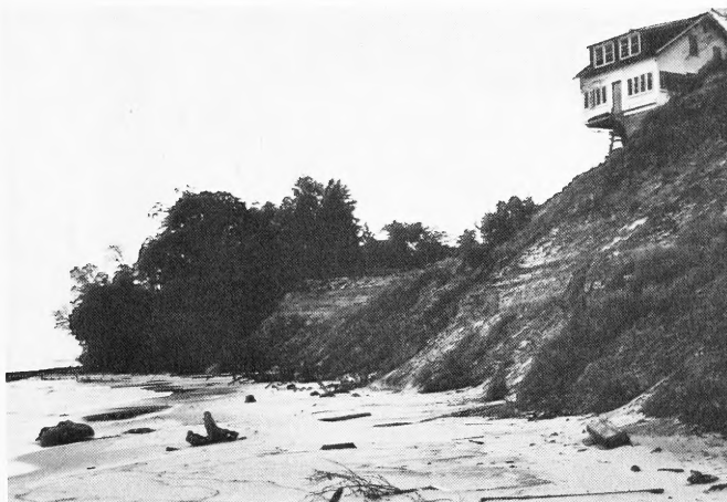
Figure 1. Severe bluff erosion undermining lakefront home near Stevensville, Michigan (17 October 1976).
