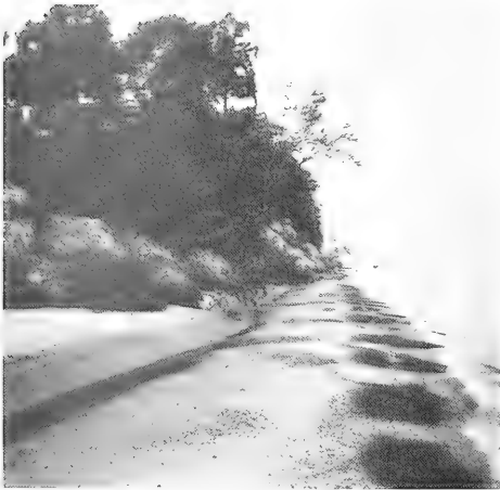
16 August 1974 - Note failing bluff line and accretionary beach ridge. Dark patches on the foreshore are periodic gravel deposits.
