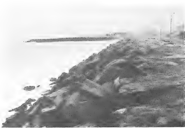
Figure 3. Seawall and groin at Sandy Hook (looking south)
