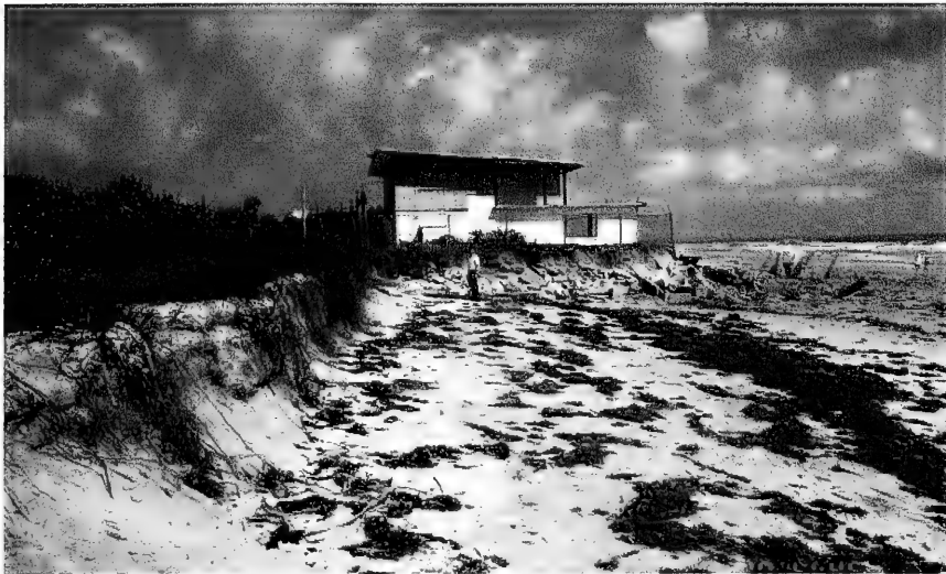
Figure 4-2. Applegate property viewed from the south adjacent property, February 20, 1997. Location of Applegate residence and rubble on the beach face and in front of the dune line is clearly evident (source: N. C. Kraus).
