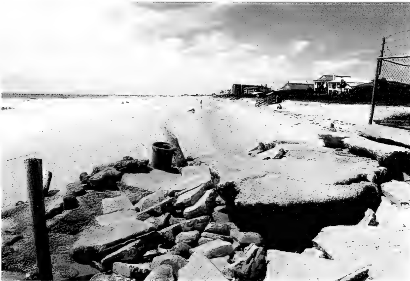
Figure D-13: View looking south from Applegate residence, May 9, 1996 (source: N. C. Kraus).
