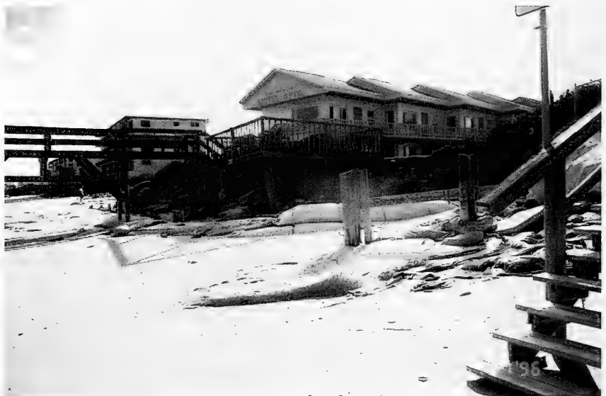
Figure D-23: Noro and Co. property, November 21, 1996, showing deteriorated wooden bulkhead, geotextile sandbags, and other remains of storm-protection structures (source: N. C. Kraus).
