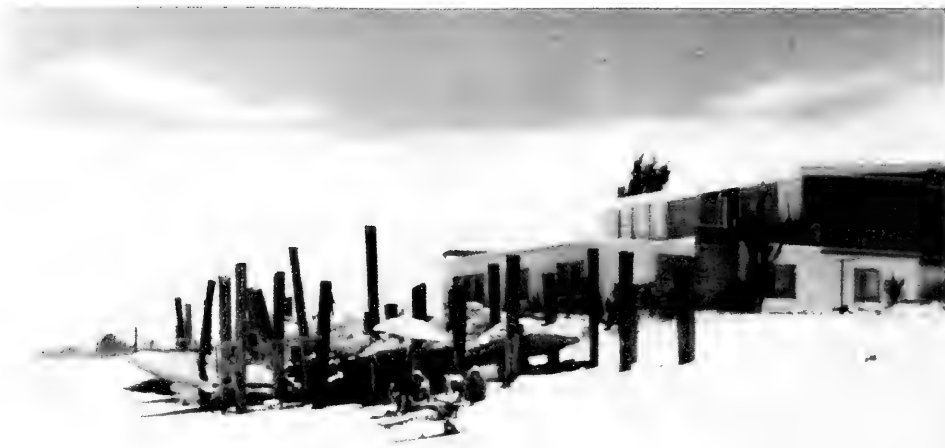
Figure D-6: Applegate property, August 1971. Presence of pilings and concrete rubble indicates this particular house was vulnerable to wave impacts soon after its construction, circa 1960 (source: USACE, Jacksonville District).
