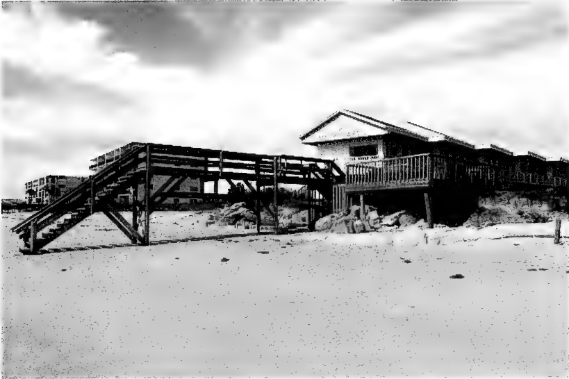
Figure D-20: Noro and Co. property, May 9, 1996. Note the old stone revetment, deteriorated wooden bulkhead, and the sandbags along the seaward side of the property under the wooden boardwalk (source: N. C. Kraus).
