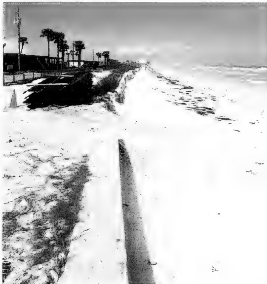
Figure D-1: View north along the concrete bulkhead at the Officers Club, Patrick AFB, February 20, 1997 (source: N. C. Kraus).
