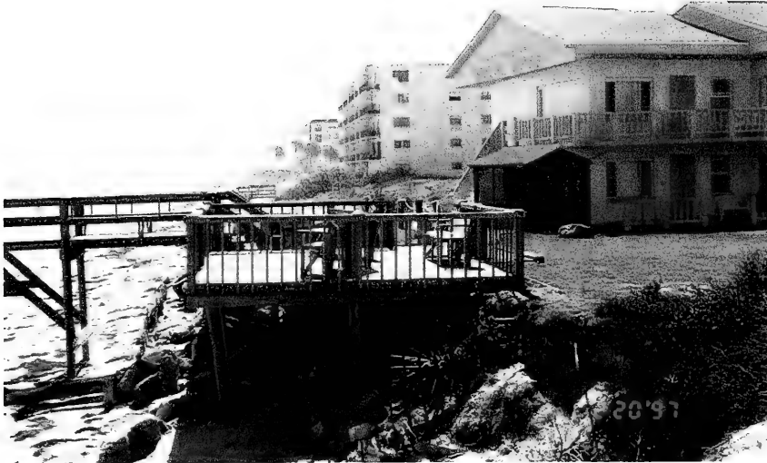
Figure D-28: Noro and Co. property, February 20, 1997. The remains of the wooden bulkhead are visible just seaward of the wooden deck ( source: N. C. Kraus).
