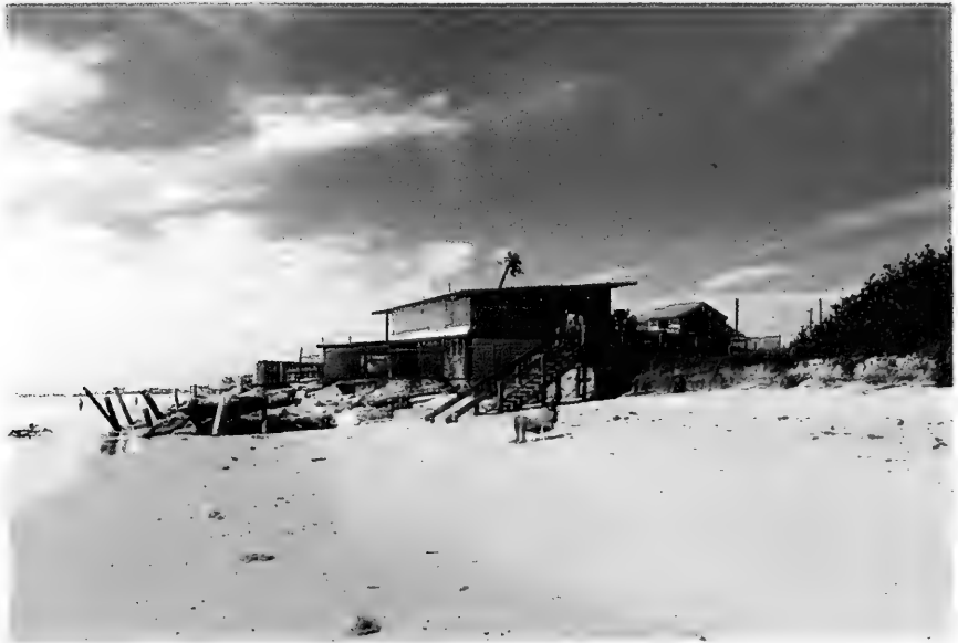
Figure D-11: Applegate property on May 9, 1996, showing location of rubble mound and structure relative to natural beach features and other structures along the coast (source: N. C. Kraus).
