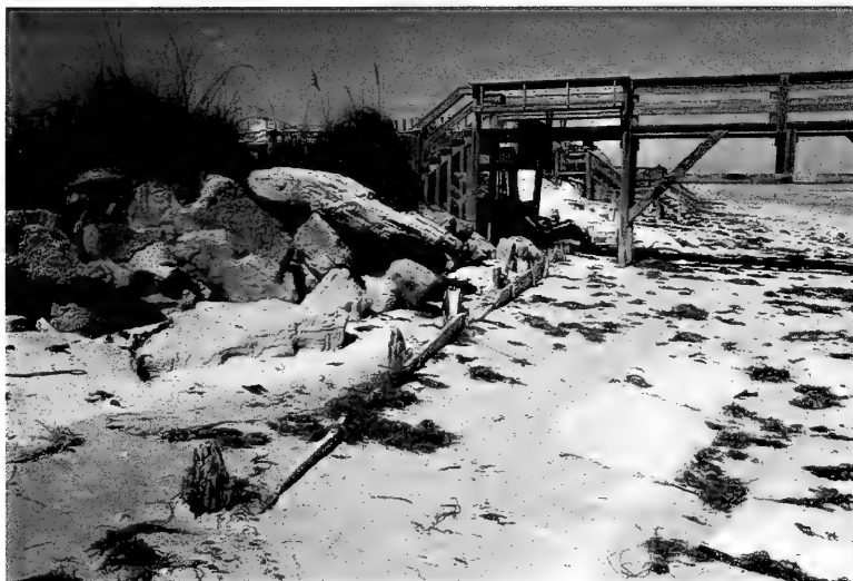
Figure 4-8. Oblique view of remnant wooden bulkhead, rock revetment, and sandbags along the seaward side of the Noro Property (Pelican Landing), February 20, 1997 (source: N. C. Kraus).
