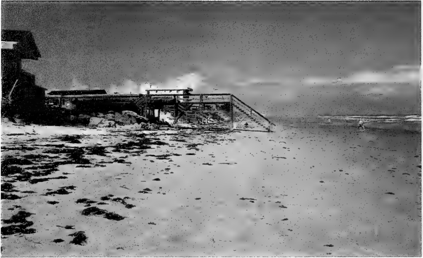
Figure 4-9. View north of Noro property with a wide beach, February 20, 1997 (source: N.C. Kraus).
