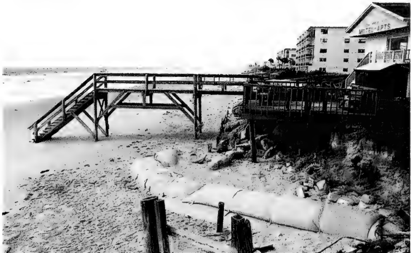
Figure 1-3. Noro and Co. property, May 9, 1996, showing the deteriorated wooden bulkhead and sandbags, as well as storm erosion at the dune face (source: N. C. Kraus).
