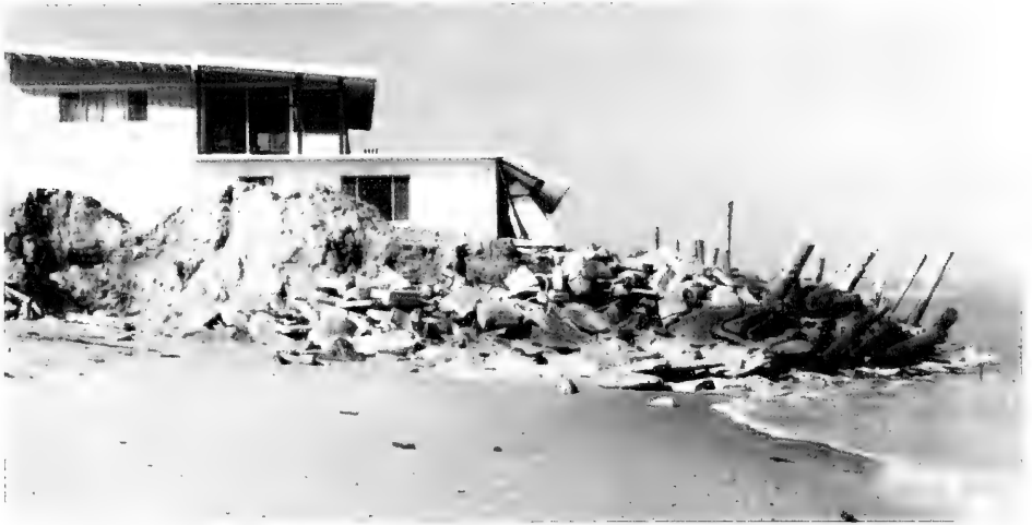
Figure D-8: South side of Applegate property between February 1973 and November 1974 (source: USACE, Jacksonville District).
