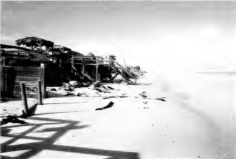
Figure D-25: View north of Noro and Co. property, November 21, 1996, showing storm damages to northern neighboring properties (source: N. C. Kraus).
