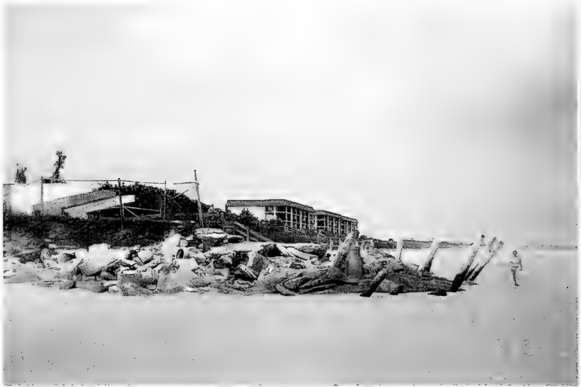
Figure 4-4. Side view of Applegate property, December 3, 1997 (source: N. C. Kraus).
