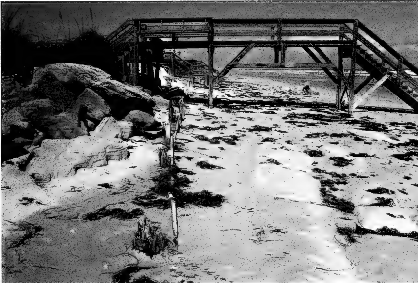
Figure D-29: View north of Noro and Co. property showing the remains of the wooden bulkhead and rock revetment, February 20, 1997( source: N. C. Kraus).
