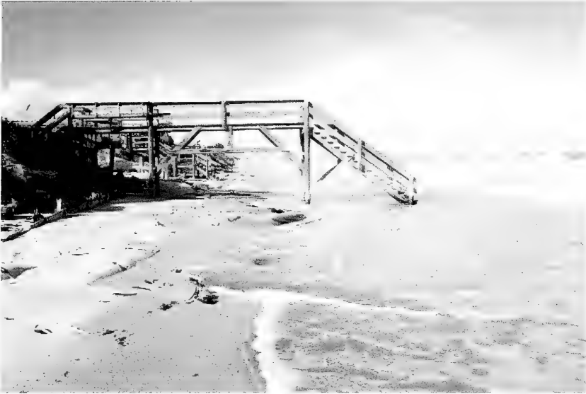
Figure D-24: View north of the boardwalk at Noro and Co. property, November 21, 1996, showing the narrow beach associated with a typical winter profile (source: N. C. Kraus).
