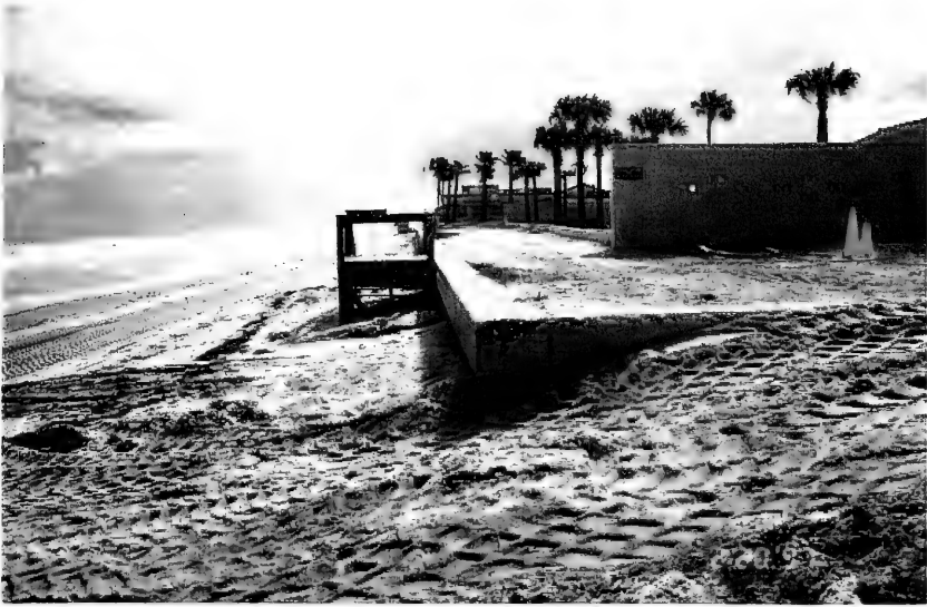
Figure 2-4. Northern end of concrete bulkhead at the Officers Club at Patrick AFB, February 20, 1997. Similar location as in Figures 2-2 and 2-3 (source: N. C. Kraus).
