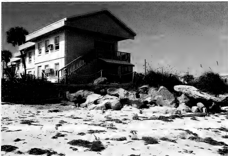
Figure 4-7. View of rock revetment and remnant wooden bulkhead seaward of the Pelican Landing Resort, February 20, 1997 (source: N. C. Kraus).
