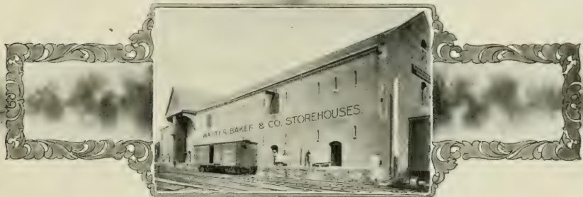
WALTER BAKER & CO.'S STOREHOUSES, MILTON.
