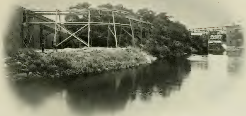
THE TELPHERAGE SYSTEM—FOR THE CONVEYANCE OF CRUDE COCOA FROM THE STOREHOUSES TO THE ROASTING ROOMS.
