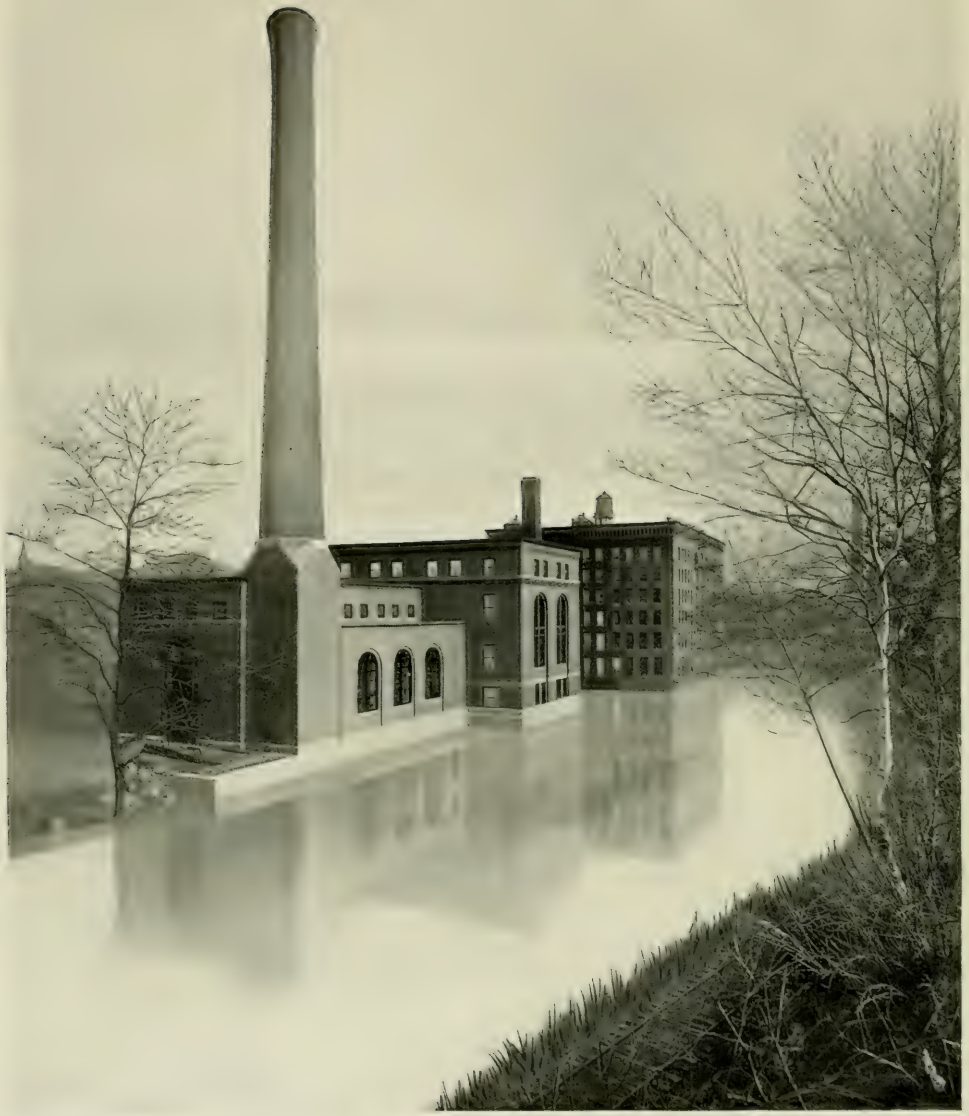
NEW POWER PLANT, 1906, WALTER BAKER & CO. LTD.
