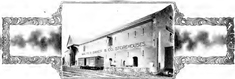
WALTER BAKER & CO.'S STOREHOUSES, MILTON.
