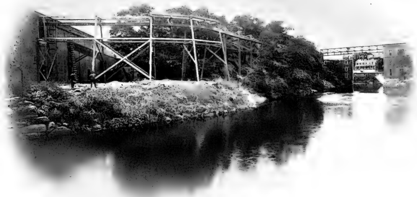
THE TELFERAGE SYSTEM — FOR THE CONVEYANCE OF CRUDE COCOA FROM THE STOREHOUSES TO THE ROASTING ROOMS.
