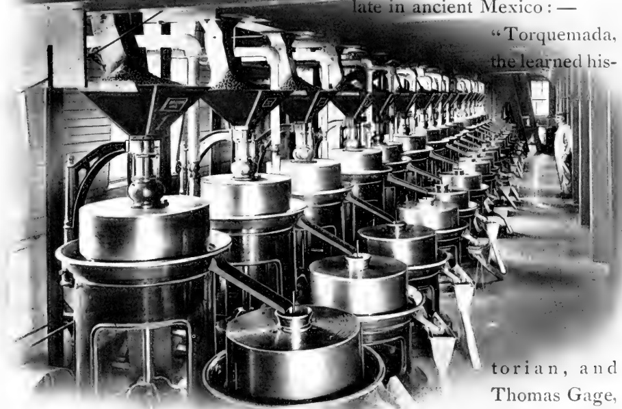
GRINDING ROOM IN ONE OF WALTER BAKER & CO.'S MILLS.
