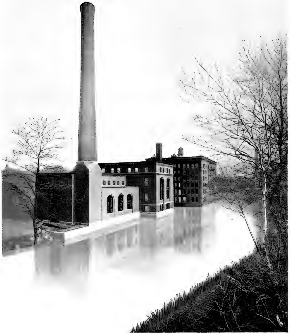
NEW POWER PLANT, 1906, WALTER BAKER & CO. LTD.
