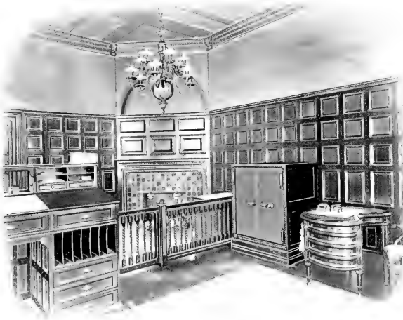
PRIVATE OFFICE, MILL NO. 4.
