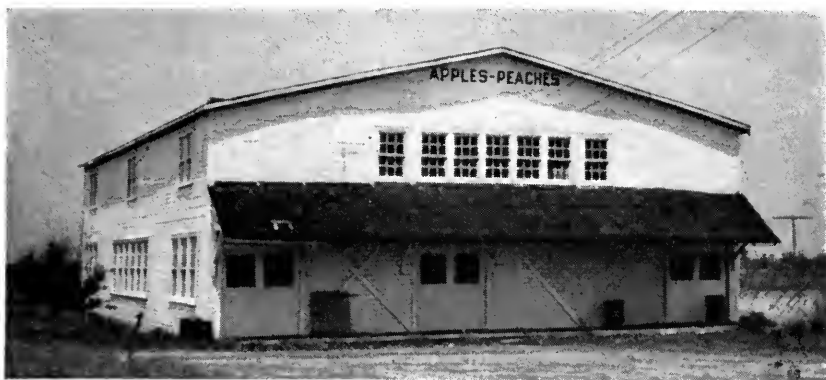
A packing shed of this type can easily be made moth-tight. Here a little battening put over the cracks kept moths, hatched out on containers in the shed, from escaping to the orchard.
