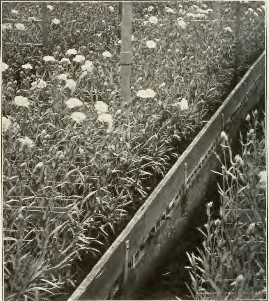
VIEW OF SIDE OF BENCH SHOWING CEMENT BASE, TILE BOTTOM AND STRONGLY BRACED WOODEN SIDE
