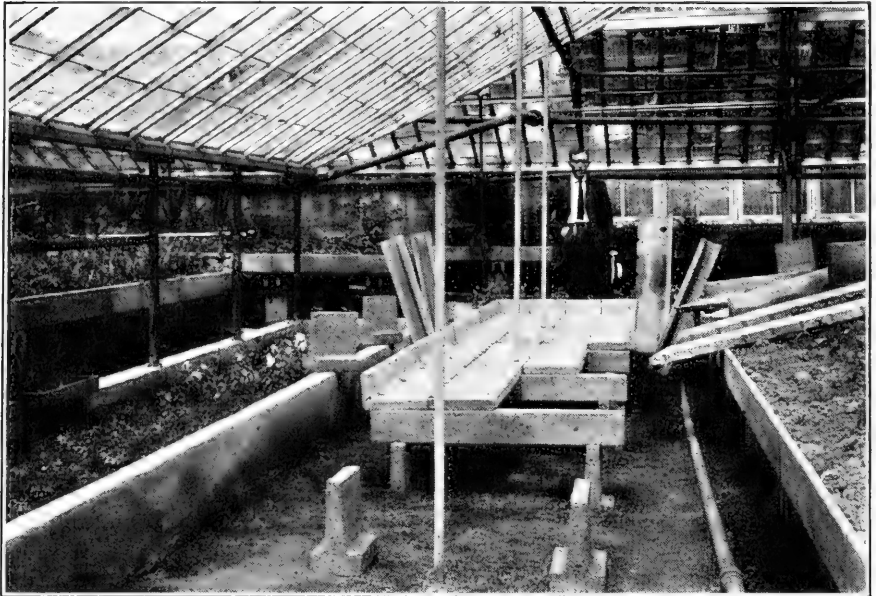
MCCASLAN'S SECTIONAL CONCRETE BENCH IN SECTIONAL SLABS
