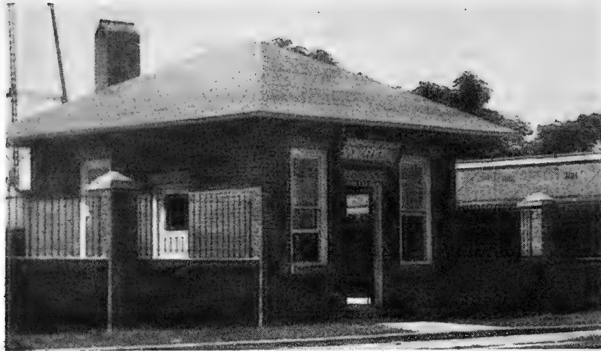
TARPON SPRINGS SPONGE EXCHANGE BUILDING
