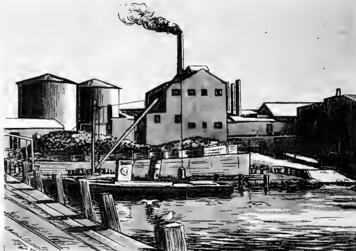
SHORE-WHALING STATION AT DONKERGAT, ONE OF TWO OPERATING IN THE UNION OF SOUTH AFRICA. THE SLIPWAY AND FLENSING STAGE ARE ON THE RIGHT, WITH THE BUILDING WHERE THE MEAT IS PROCESSED ON THE EXTREME RIGHT. THE BLUBBER IS BOILED DOWN IN THE CENTER BUILDING, AND THE OIL STORED IN TWO TANKS ON THE LEFT.
