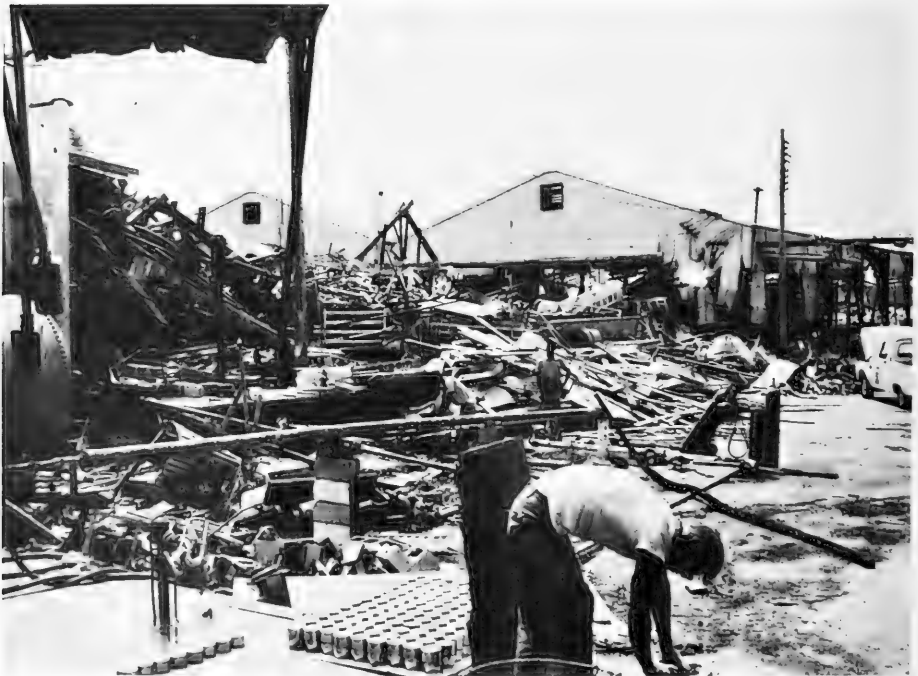
Fig. 3 - Cleanup begins in Biloxi.
