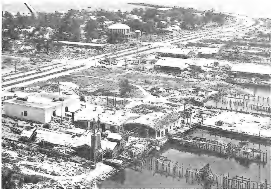
Fig. 1 - Aerial view of "Cannery Row" Biloxi after hurricane Camille.
