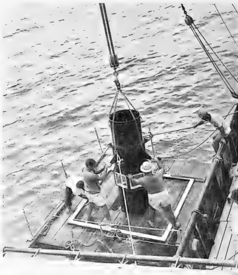
The underwater caisson being lowered on to the Nenu I from the mothership, Charles H. Gilbert .
