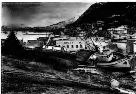
Fig. 3 - Part of the downtown section of Kodiak after the earthquake. Note how vessels were tossed onto the land.
