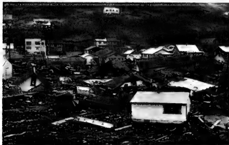
Fig. 2 - Viewing upper downtown section of Kodiak from a hillside. About 24 dwellings were demolished, and many others were moved as much as 4 blocks off their foundations. A good part of the business district sustained substantial damage.
