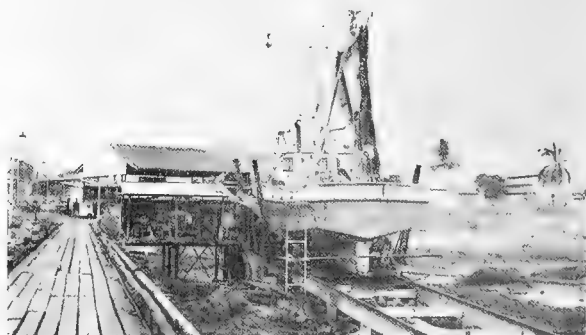
Fig. 3 - This shrimp firm in Panama City has its own fleet, and marine ways for repair of both its own fleet and independent vessels that fish for the plant.
