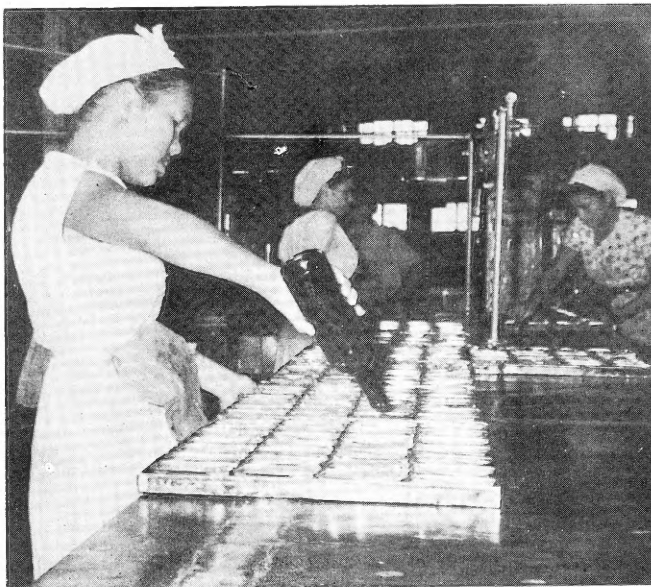
ADDING OIL TO SARDINES (FOREGROUND) AND SEALING THE CANS (BACKGROUND)
