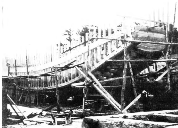
FIGURE 2 - THE FRAMEWORK OF A JAPANESE TUNA BOAT.
