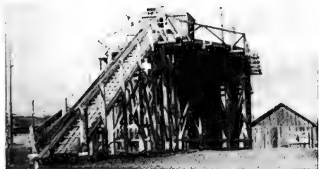
Fig. 4 - Fish conveyor under construction, Ohkotsk Combine.
