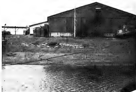
Fig. 28 - Cold storage at October Combine as seen from the river.
