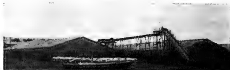
Fig. 23 - Fish-delivery conveyor to processing plant, October Combine, Kamchatka.
