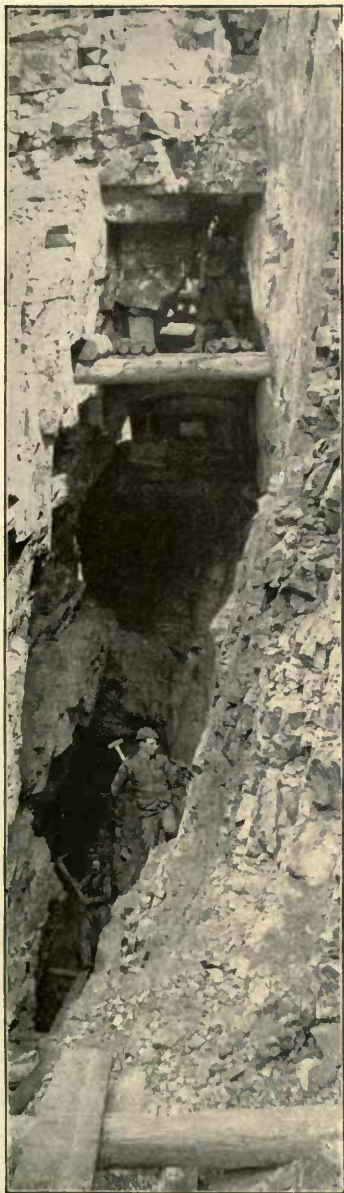
STOPING OUT A TUNNEL
