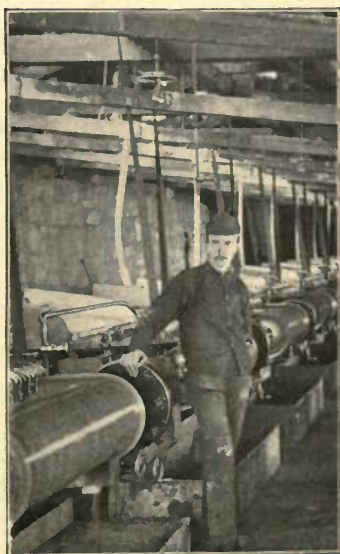
INTERIOR OF MILL
