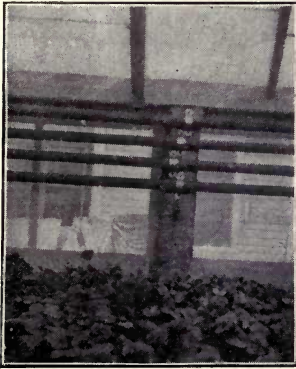
14.—Fastening pipes to posts by tin clips.
