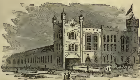
ILLINOIS CENTRAL RAILROAD DEPOT, CHICAGO.
