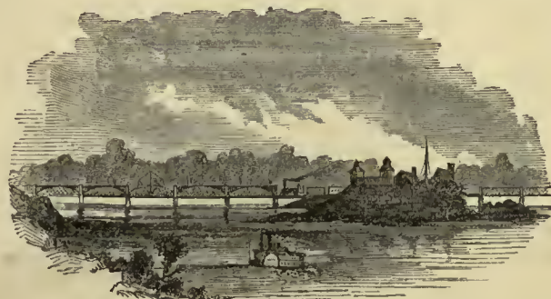
BRIDGE ACROSS THE MISSISSIPPI RIVER, AT ROCK ISLAND.
