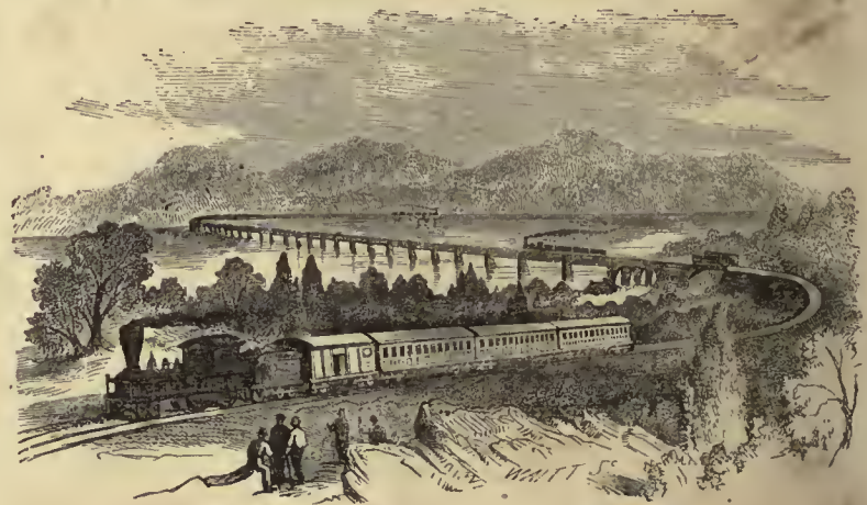
PENNSYLVANIA RAILROAD BRIDGE, ACROSS THE SUSQUEHANNA RIVER.
