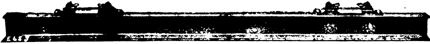
THE U.S. STEEL TIE WITH TIE RAIL FASTENINGS BEFORE THE CONCRETE IS MOULDED AROUND IT.
