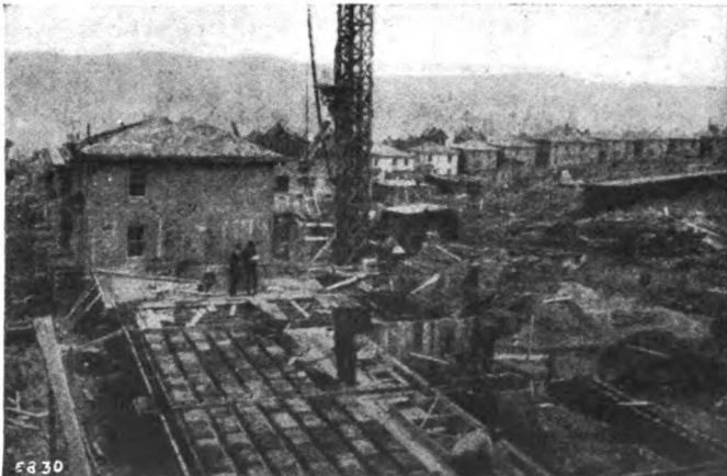
Method of spouting concrete from tower. CONCRETE DWELLINGS SCHEME IN U.S.A.
