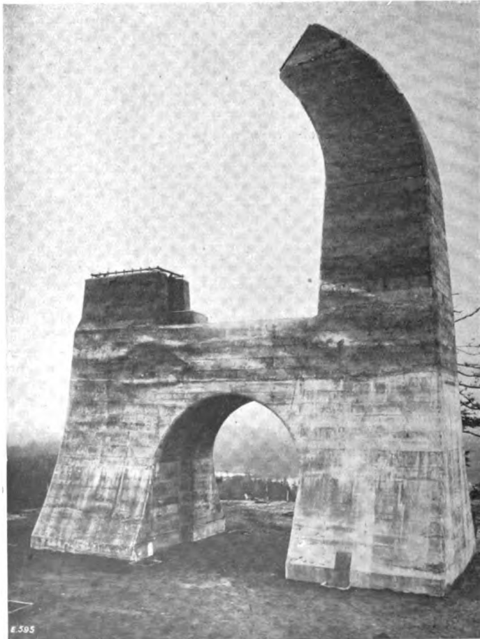
VIEW SHOWING CONCRETE CONSTRUCTION TOWER FOR TELESCOPE AT MOUNT SAANICH, B.C.
