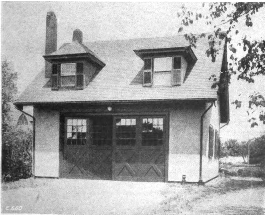
Fig. 11. A concrete garage with living quarters above.
