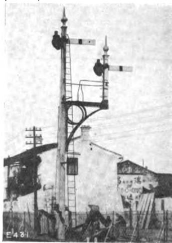
FIG. 9. A CONCRETE BRACKET SIGNAL ON A CHINESE RAILWAY.
