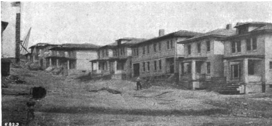
Some of the houses nearly completed. CONCRETE DWELLINGS SCHEME IN U.S.A.
