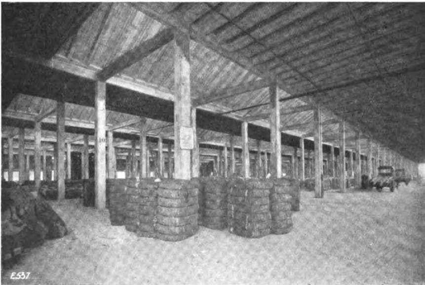
Fig. 11. Interior of Compress Room. REINFORCED CONCRETE CONSTRUCTION IN THE NEW COTTON WAREHOUSES AND TERMINALS OF THE PORT OF NEW ORLEANS.
