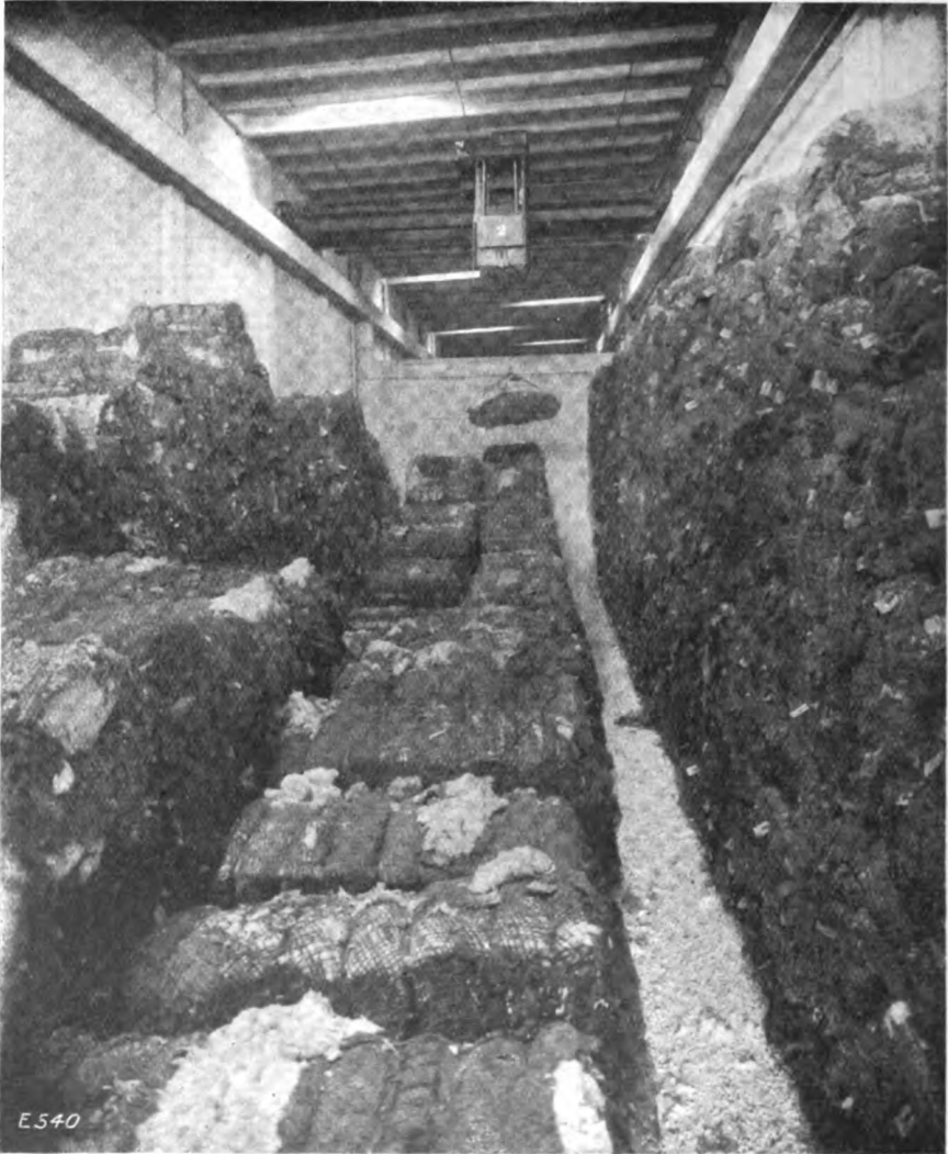
Fig. 9. Interior of Typical Warehouse Compartment.
