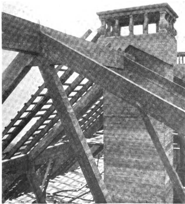
Fig. 9. Reinforced Concrete roof construction.
