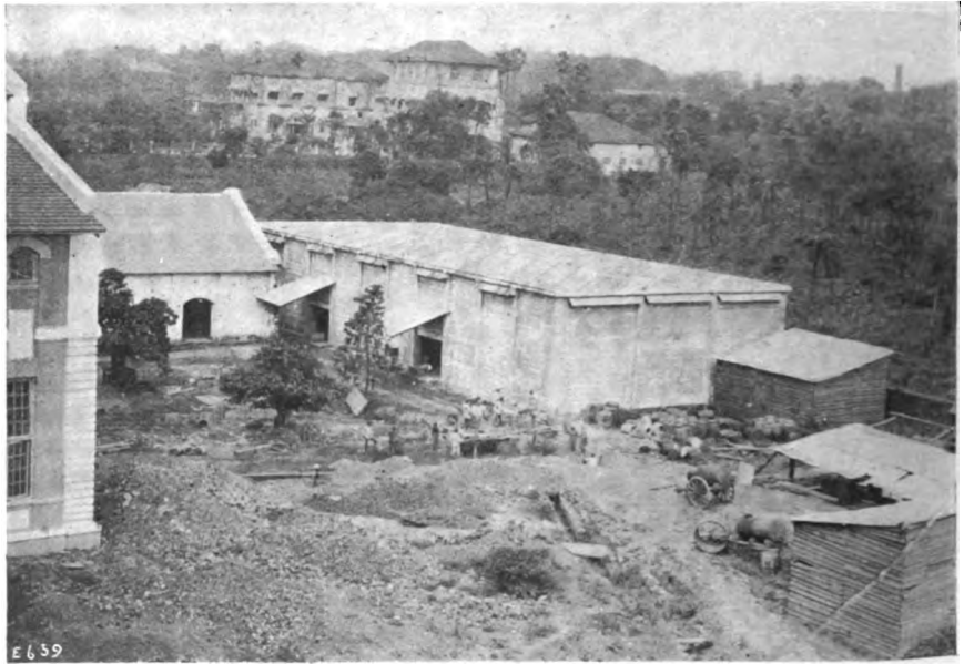
Fig. 3. Illustrating another example of the type of Roof shown in Fig 2. REINFORCED CONCRETE ROOFS IN INDIA.
