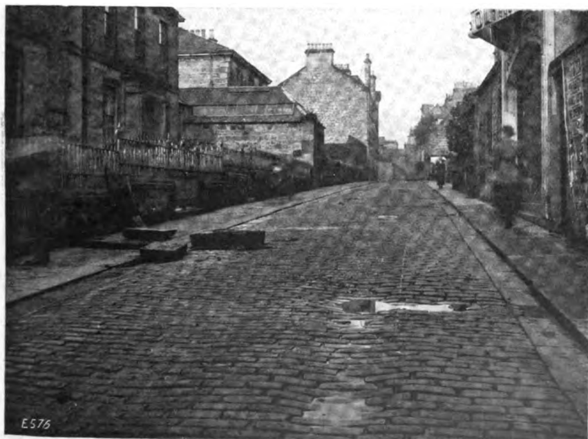
Fig. 1. Road Prior to Reconstruction. REINFORCED CONCRETE STREET WORK IN CANMORE STREET, DUNFERMLINE.
