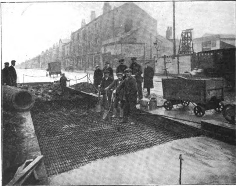
Johnson's Steel Wire Lattice for all classes of Road Reinforcement.
