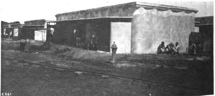
Figs. 5 & 6. A view of part of Khargpur Village. Showing Artisans' Dwellings cast 'en bloc' in Concrete. REINFORCED CONCRETE ROOFS IN INDIA.
