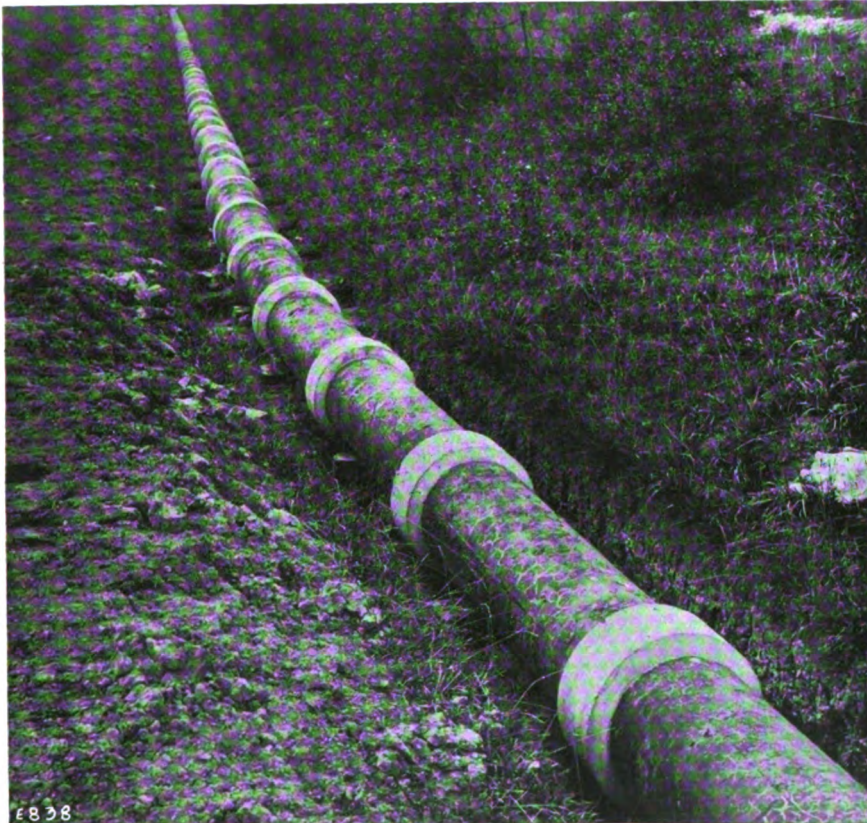
14-IN. DIA. REINFORCED CONCRETE GAS MAINS FOR THE BARNSELY SMOKELESS FUEL CO.
