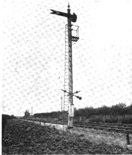
FIG. 11. A SLOTTED DISTANT SIGNAL POST AS USED ON THE MIDLAND RAILWAY.
