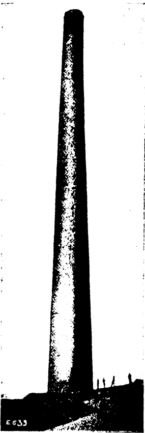
A REINFORCED CONCRETE CHIMNEY IN JAPAN.
