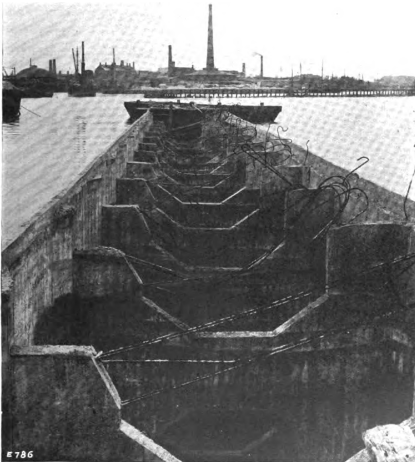
FIG. 6. REINFORCED CONCRETE CAISSON, IN COURSE OF CONSTRUCTION, AT COPENHAGEN.
