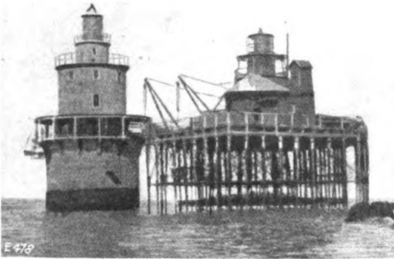
THE NEW REINFORCED LIGHTHOUSE AND THE OLD IRON LIGHTHOUSE. BRANDYWINE SHOAL, U.S.A.
