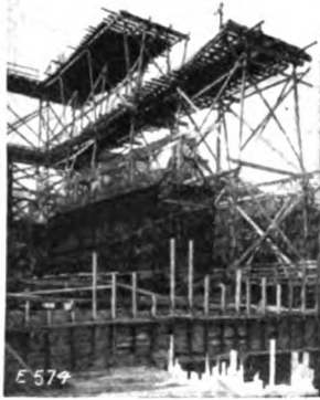
TURBINE HOUSE IN COURSE OF ERECTION.
