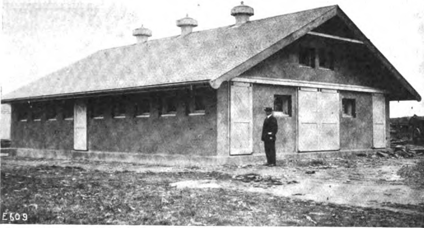
FIG. 3. A CONCRETE COW STABLE. EXTERIOR VIEW.
