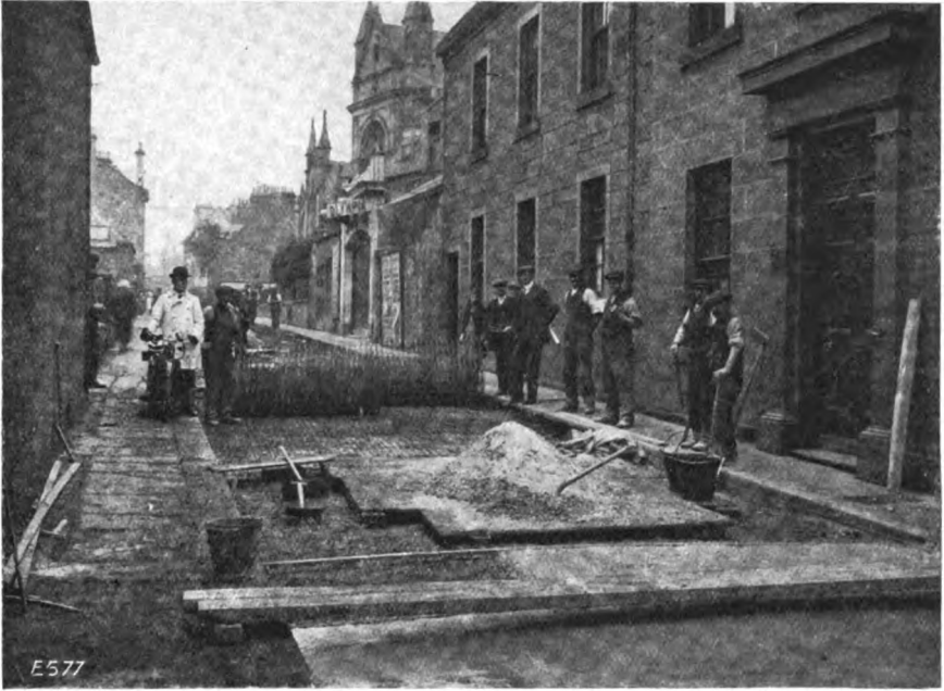
Fig. 2. Road during construction.
