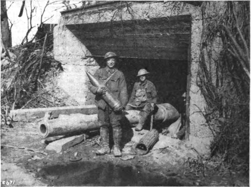
AN EXAMPLE OF A GERMAN CONCRETE EMPLACEMENT.—A CAPTURED 8-IN. NAVAL GUN IN ITS EMPLACEMENT AT FARBUS.
