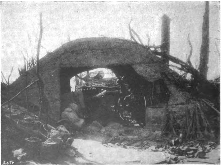
ANOTHER TYPE OF CONCRETE EMPLACEMENT BUILT ABOVE GROUND.—A GERMAN GUN CAPTURED BY THE CANADIANS IN FARBUS WOOD.
