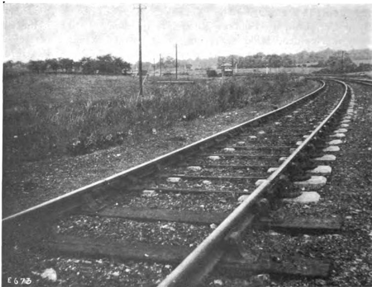
VIEW OF THE YOKEBLOCK CONCRETE SLEEPER AT NEASDEN BY J. ALLEN.
