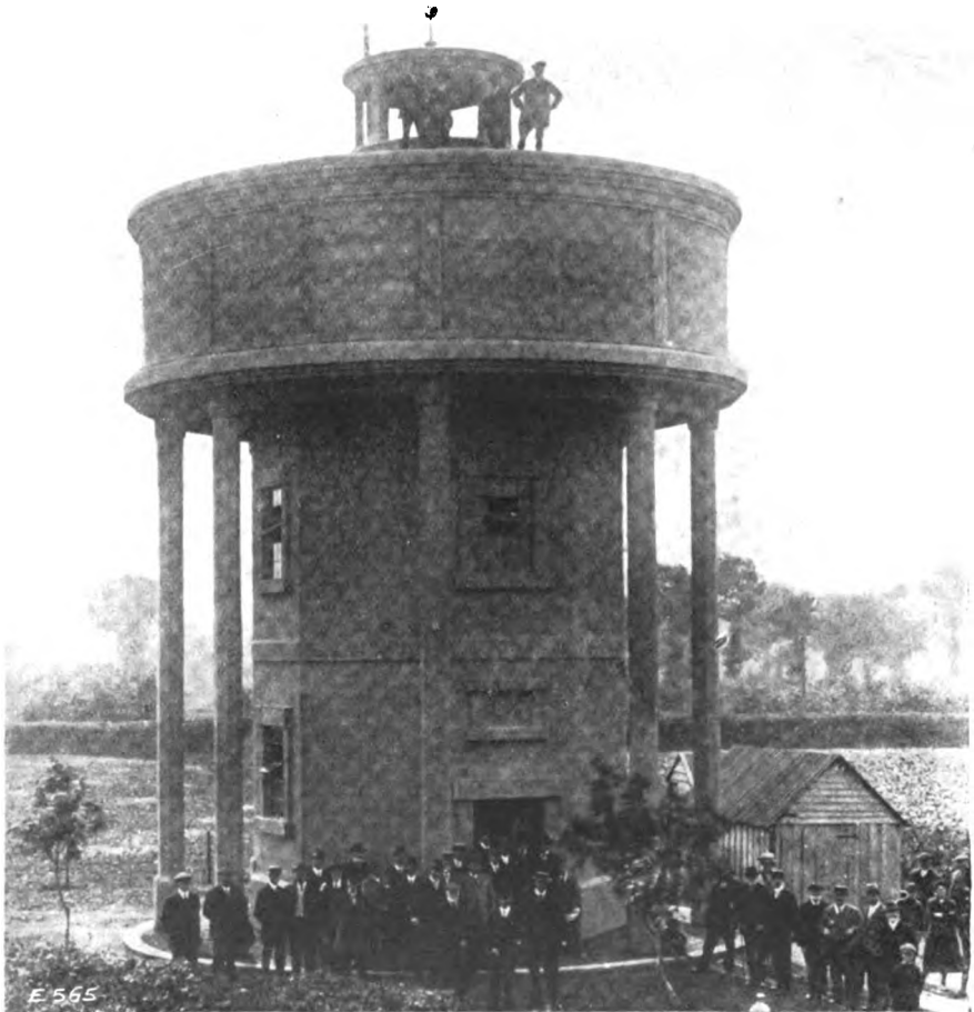
Finished View of Structure.
