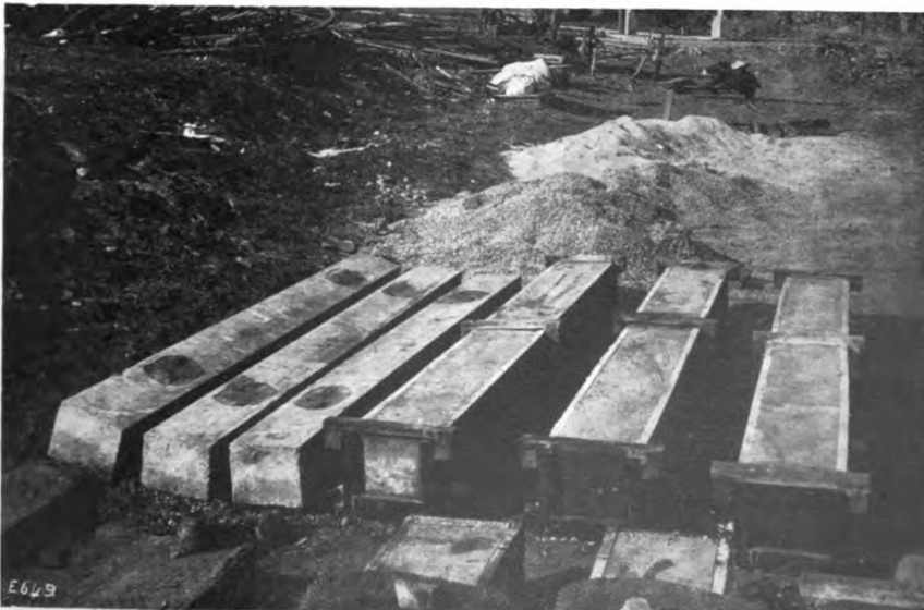
THE TIE PREPARED FOR THE SANTA FE RAILROAD, LOS ANGELES, CALIFORNIA.
