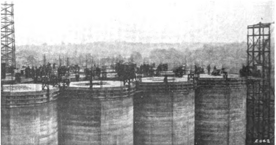
Fig. 9. Showing Centering for Silos. NEW NUT SILOS AND WAREHOUSES.
