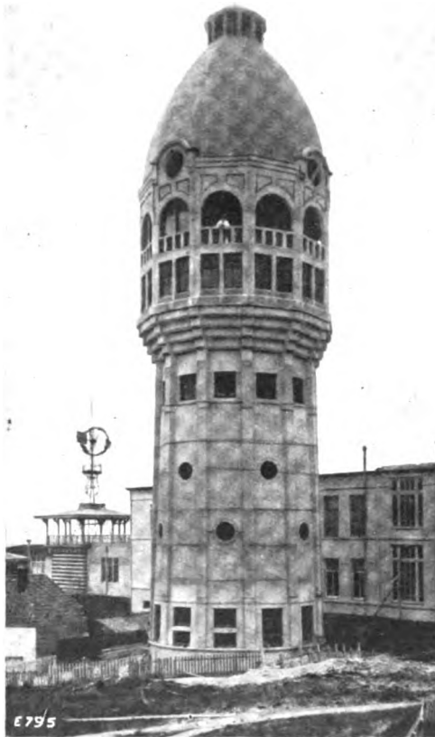
Fig. 10. Water Tower at Zandvoort. REINFORCED CONCRETE WATER TOWERS IN HOLLAND.
