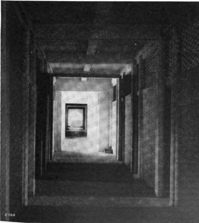
View of Passage dividing the double row of rooms. REINFORCED CONCRETE CHAWLS FOR MILL WORKERS IN INDIA, AT SPRING MILLS, NAIGAUM ROAD, DADAR, NR. BOMBAY.
