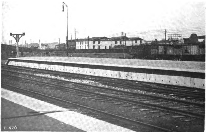
FIG. 14. CONCRETE PLATFORM WALL BLOCKS IN POSITION.
