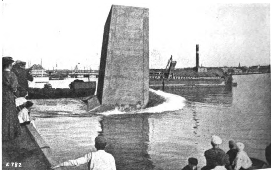
FIG. 7. REINFORCED CONCRETE CAISSON BEING LAUNCHED AT NORRESUNDEY, DENMARK.
