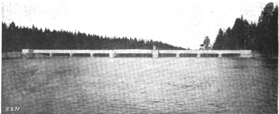
Fig. 11. The Dam at Kingsdra Falls.
