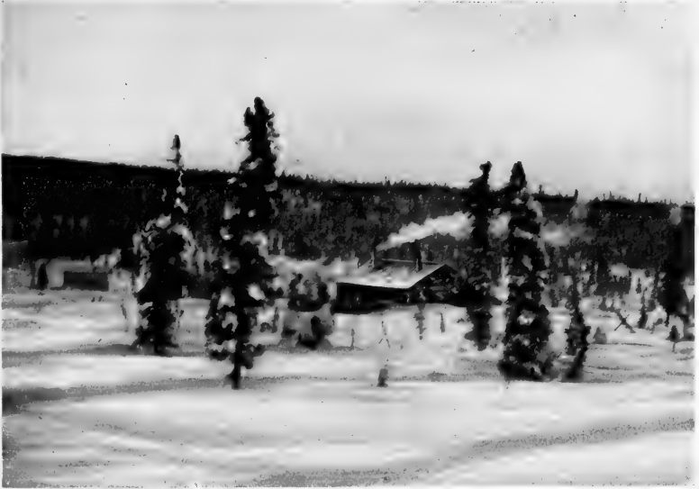
" OUR HOME " ( A ROAD-HOUSE ).
