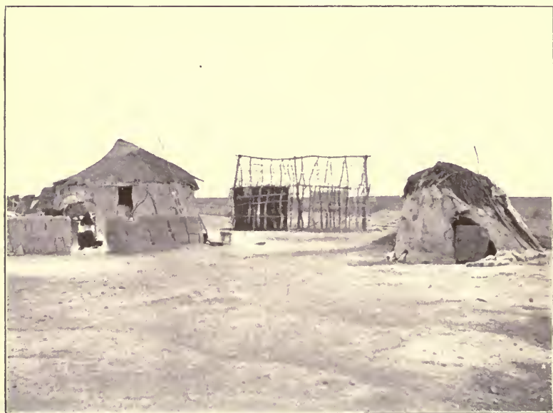
(FIG. 2.) A BUILDING BOOM IN THE MAIN STREET OF RIETFONTEIN, GORDONIA.
