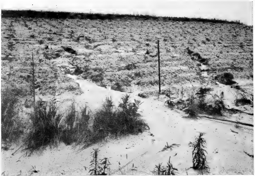
FIGURE 17.—Special attention should be given low places in tobacco fields. Lack of adequate grade in these tobacco rows has caused serious damage.
