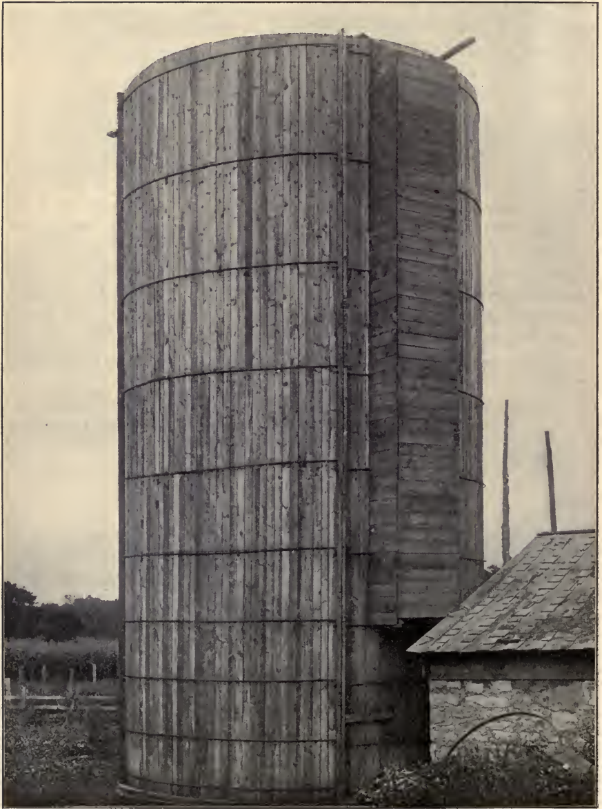
CUT 32.—STAVE SILO WITHOUT ROOF, 16 FEET IN DIAMETER AND 34 FEET DEEP; CAPACITY 150 TONS. TO BE RECOMMENDED ONLY WHERE A TEMPORARY SILO IS DESIRED.
