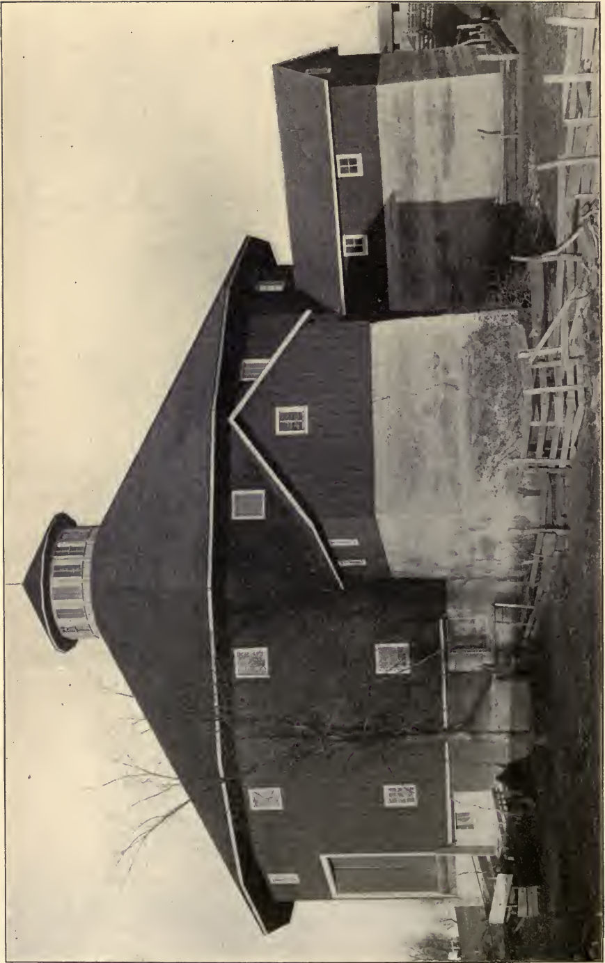
CUT 10.—SQUARE CEMENT SILOS CONNECTED WITH BARN. NOT PROPER SHAPE AND TOO SHALLOW.
