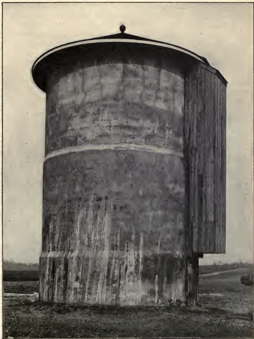
CUT 28.—CONCRETE SILO 20 FEET IN DIAMETER AND 42 FEET DEEP; CAPACITY 334 TONS.
