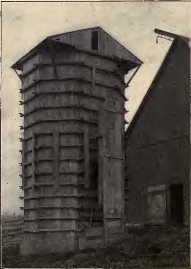
CUT 9.—CHEAP OCTAGONAL SILO WHICH DID NOT PRESERVE ITS CONTENTS PERFECTLY. THIS IS NOT A GOOD SHAPE EVEN WHEN PROPERLY CONSTRUCTED.
