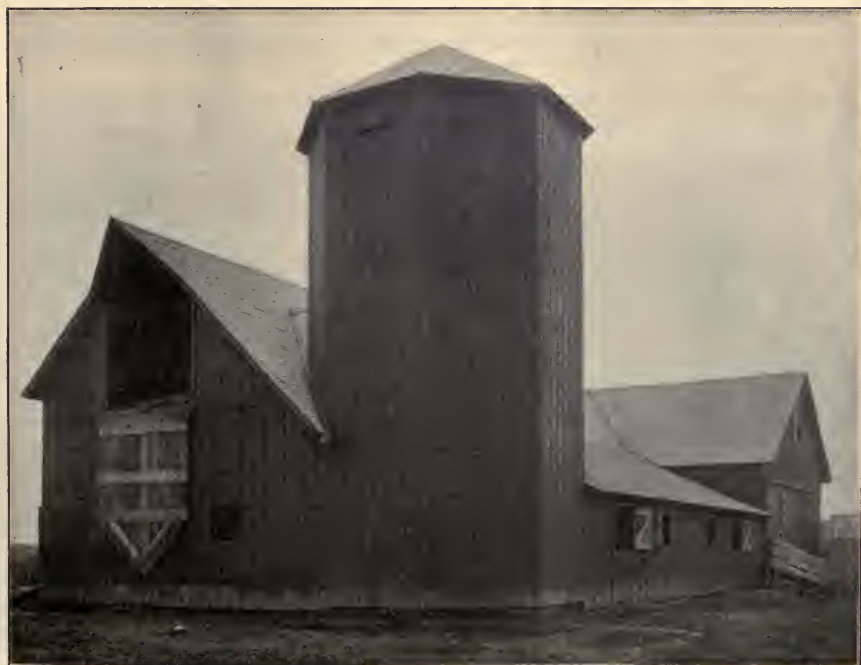
CUT 4 —OCTAGONAL SILO LOCATED IN CORNER OF BARN.
