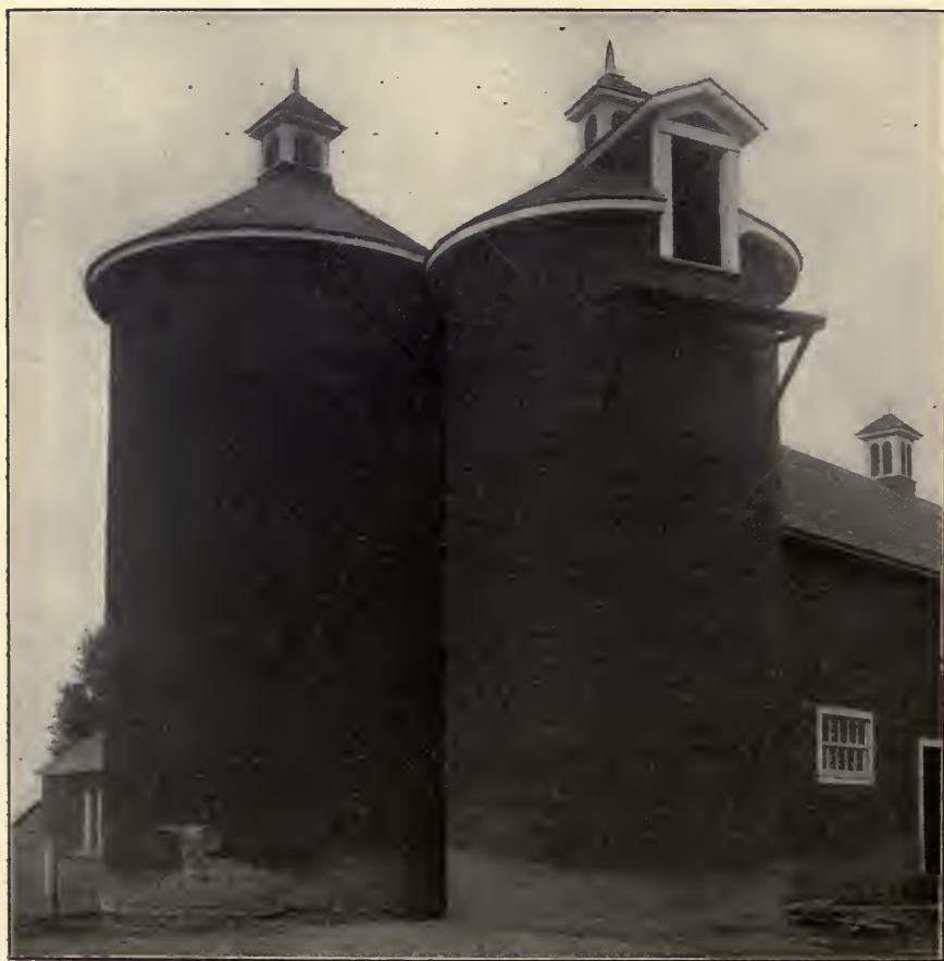
CUT 24.—TWO SILOS OF SAME CONSTRUCTION AS SHOWN IN CUT 22, SHEETED WITH HALF-INCH LUMBER; ONE ON LEFT ALSO COVERED WITH TAR PAPER.
