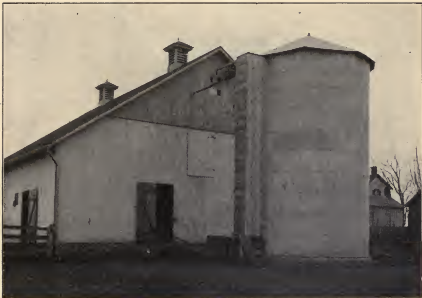
CUT 7.—WHERE NECESSARY TO FILL HAY LOFT FROM END OF BARN AT WHICH SILO IS LOCATED, A MOVABLE TRACK AND CAR MAY BE USED TO CARRY SILAGE TO MANGER.
