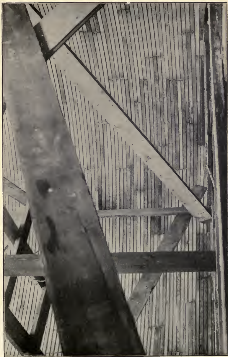
CUT 18.—INTERIOR OF SILO SHOWING LATH AND STAGING.
