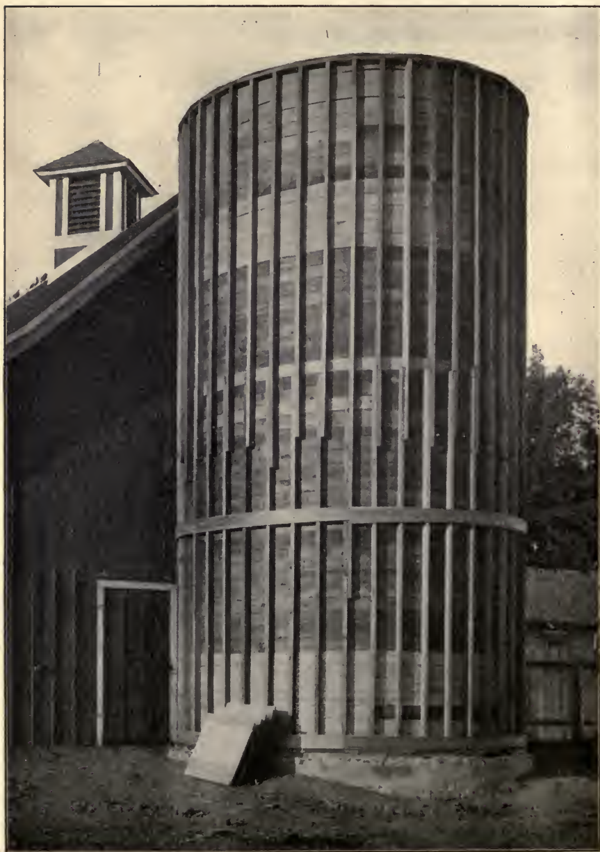
CUT 22.—SILO CEILED ON THE INSIDE WITH TWO THICKNESSES OF HALF-INCH LUMBER WITH PAPER BETWEEN. BARN WAS BUILT OVER SILO LATER.
