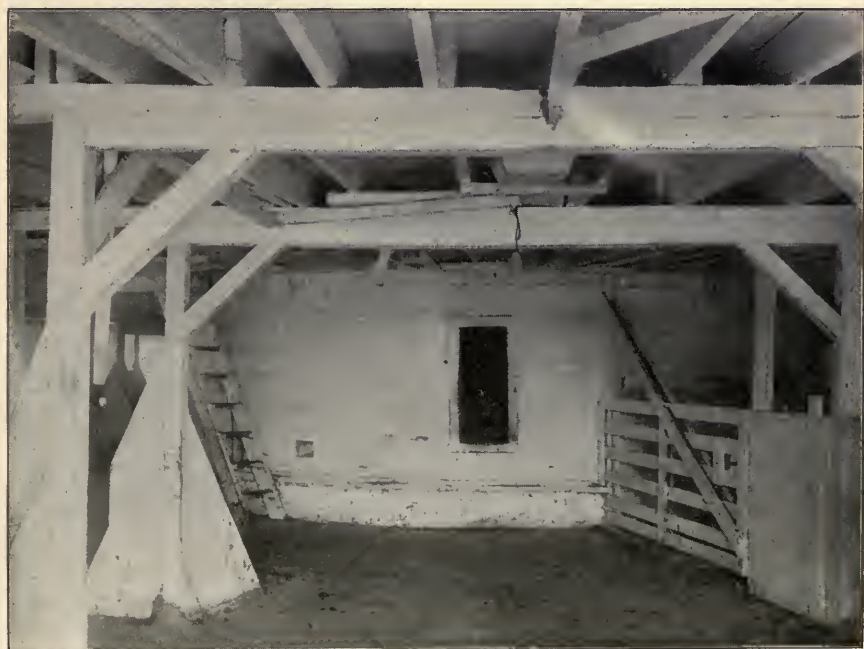
CUT 27.—SILO IN CENTER OF BARN SHOWN IN CUT 26. UPPER PORTION IN HAY LOFT, LOWER PORTION IN COW STABLE.
