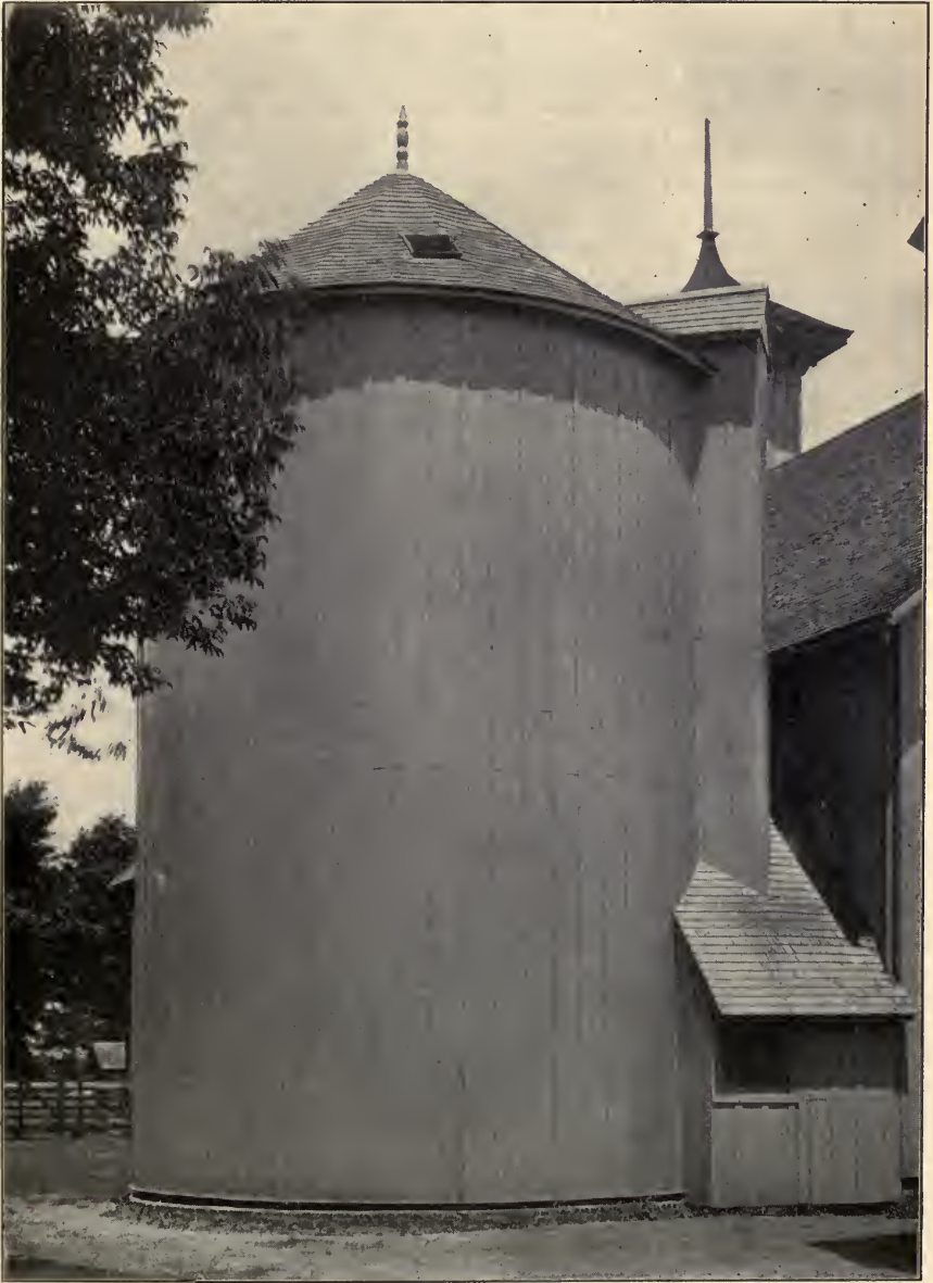
CUT 21.—THE SILO COMPLETE, SHOWING CHUTE THROUGH WHICH THE SILAGE IS THROWN DOWN, AND CONNECTION WITH THE BARN. THE SMALL DOOR IN THE ROOF IS TO ADMIT BLOWER PIPE WHILE FILLING.
