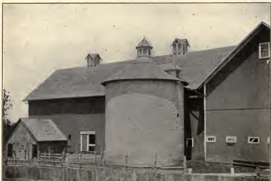
CUT 31.—STONE SILO 20 FEET IN DIAMETER AND 32 FEET DEEP; CAPACITY 204 TONS. COST NEARLY $700.
