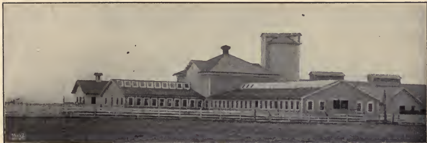
CUT 3.—SILO LOCATED AT INTERSECTION OF COW STABLES.
