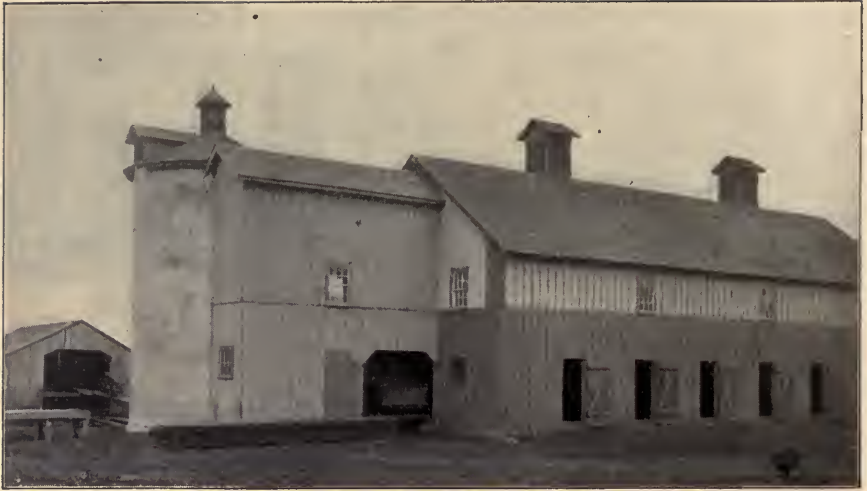
CUT 5.—SHOWING CONNECTION OF SILO WITH BARN.
