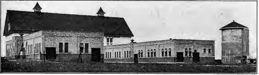
CUT 1.—LARGE CEMENT SILO TO WHICH COW STABLE IS TO BE EXTENDED.
