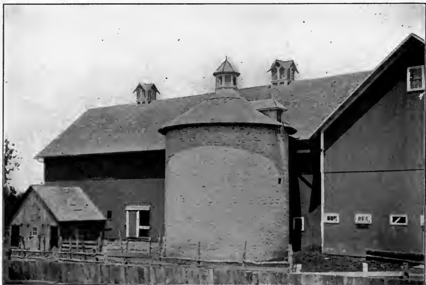
CUT 31.—STONE SILO 20 FEET IN DIAMETER AND 32 FEET DEEP; CAPACITY 204 TONS. COST NEARLY $700.
