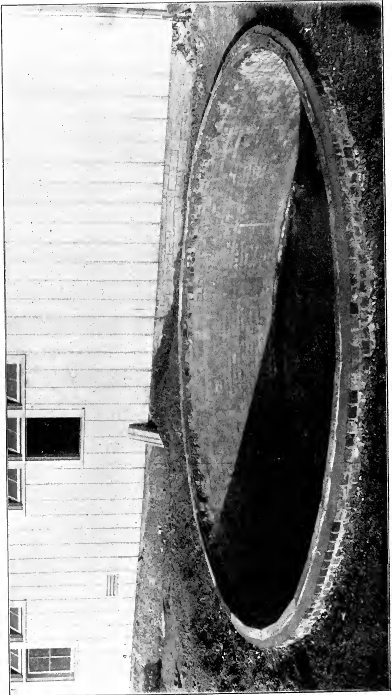
CUT II.—BRICK FOUNDATION 4¼ FEET DEEP, 2X4 SILL IMBEDDED IN CEMENT ON TOP.
