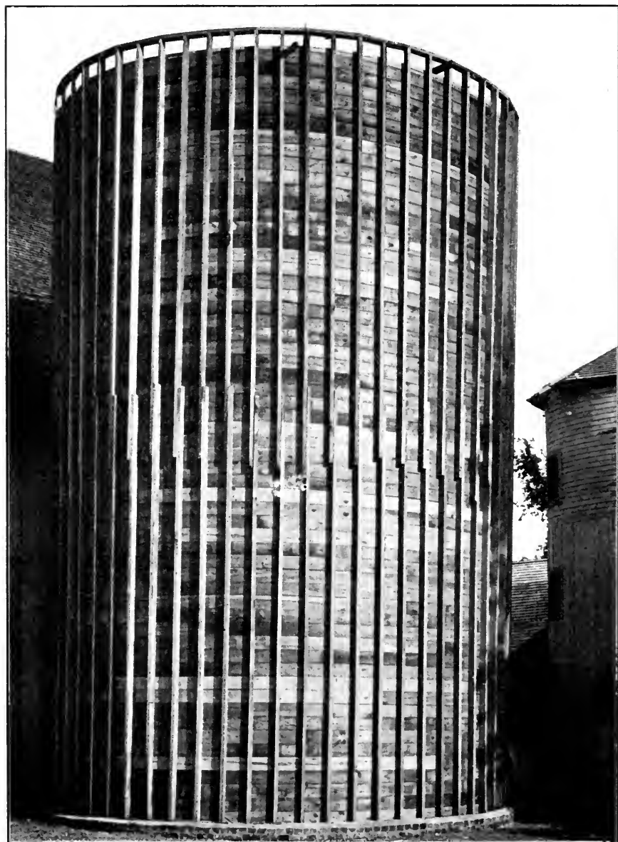
CUT 15.—INSIDE CEILING COMPLETED. CONDITION IN WHICH THE SILO STOOD FOR SIX WEEKS AFTER FILLING.
