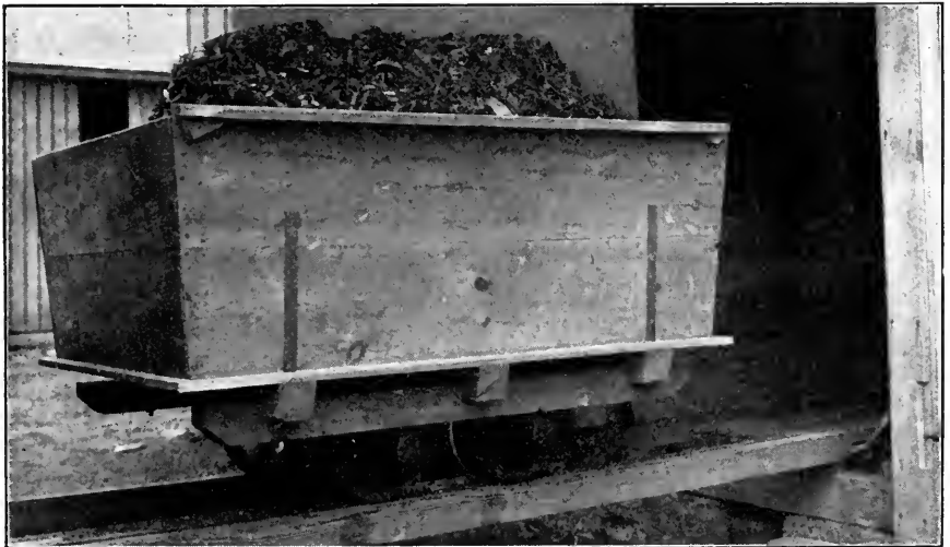
CUT 8.—SILAGE CAR TO RUN ON MOVABLE TRACK.
