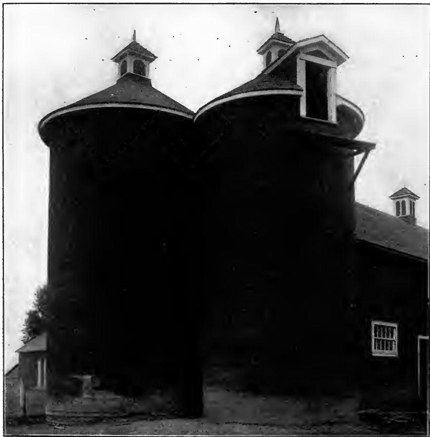
CUT 24.—TWO SILOS OF SAME CONSTRUCTION AS SHOWN IN CUT 22, SHEETED WITH HALF-INCH LUMBER; ONE ON LEFT ALSO COVERED WITH TAR PAPER.
