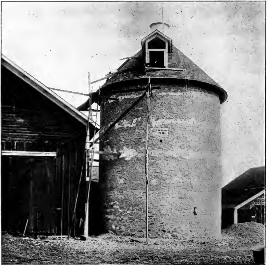
CUT 30.—STONE SILO 18 FEET 10 INCHES IN DIAMETER AND 30 FEET DEEP; CAPACITY 156 TONS. COST ABOUT $600
