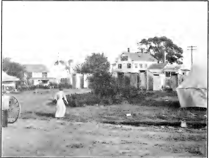
Two more views showing the construction of the privies and the proximity to the tents and cottages. (The distance is much shorter than it would seem from the pictures.)
