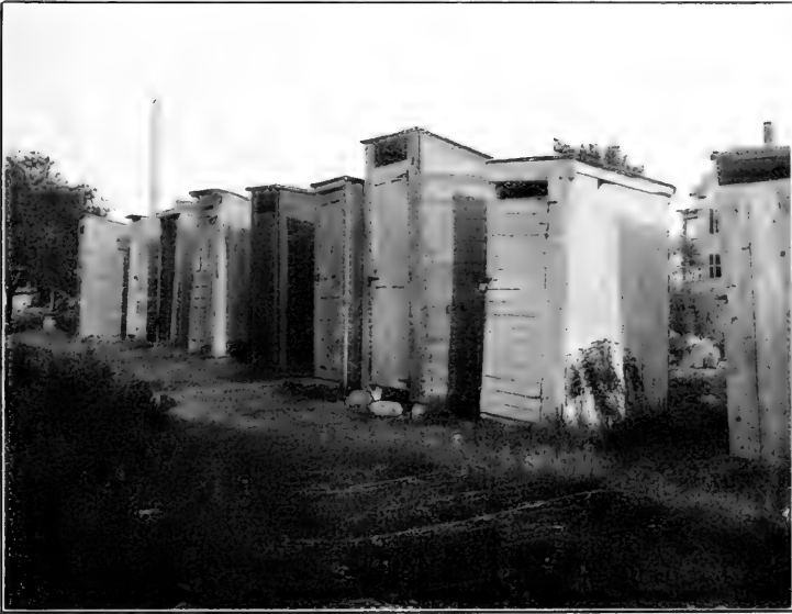
Showing the construction and "ventilation" of the privies. Note the wide open spaces under the bottom and over the tops of the doors.
