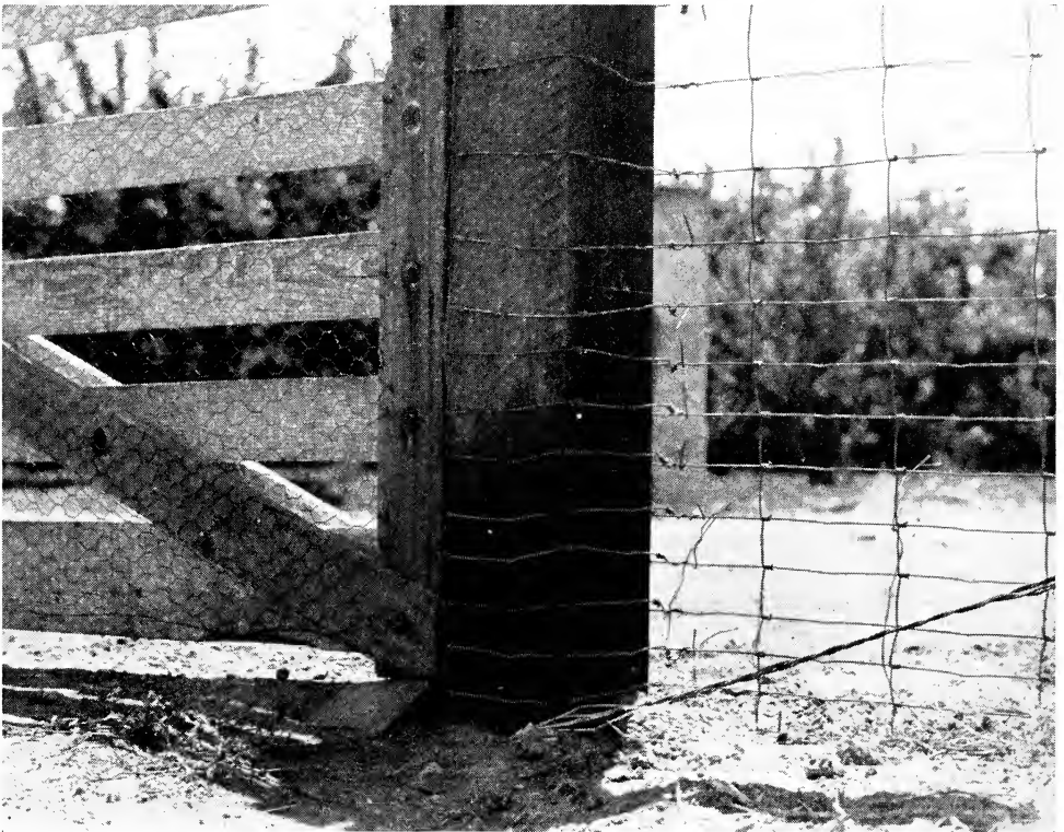
Fig. 25. Rabbitproof fence and gate. Bottom of fence wire is buried 6 inches or more and lower meshes should not be more than 1½ inches apart. Gate is covered with 1-inch poultry netting and bottom of gate must be within 1½ to 2 inches of the ground.
