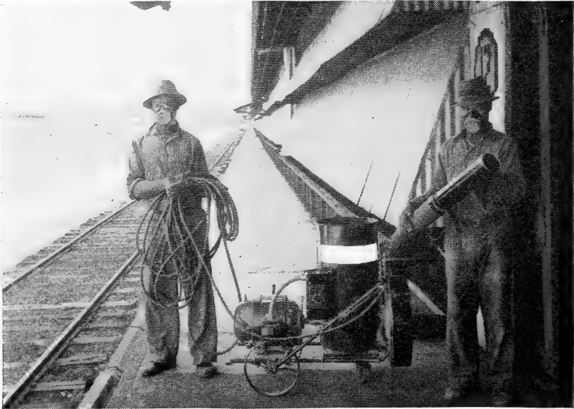
FIGURE 15.—Power duster for applying pyrethrum powder, with operating crew and equipment for dusting open warehouses.
