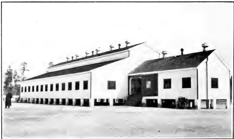
FIG. 2.—PERMANENT FRAME QUARTERS OF GOOD DESIGN.
