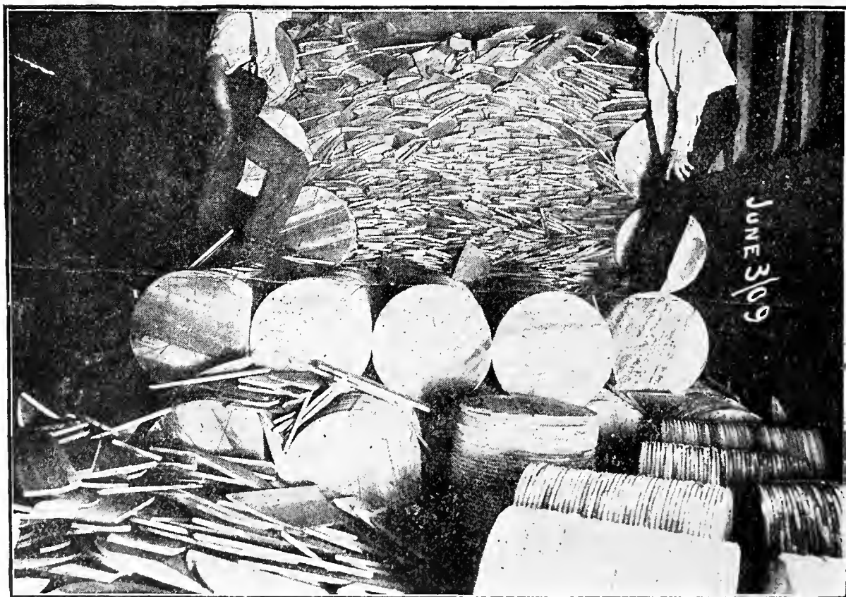
FIG. 91. VIEW SHOWING RESULTS OF POOR BUNDLING.
