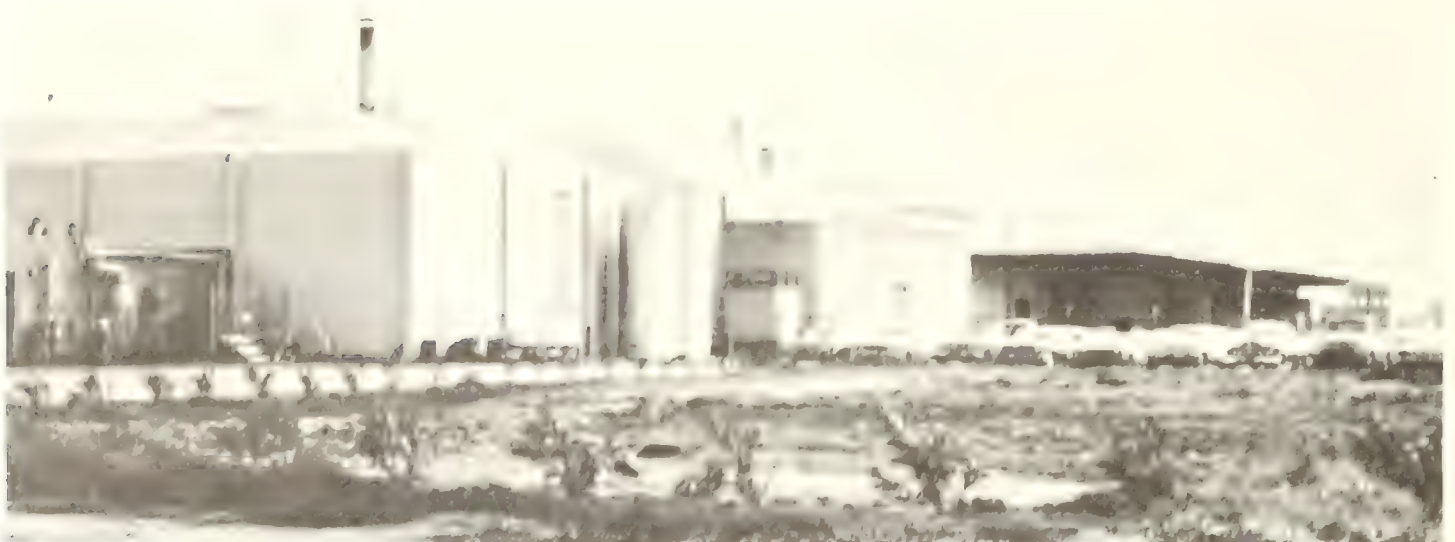
Plant of CT Supply Co., Fremont, Calif., is a one-story concrete building covering about 200,000 square feet.
