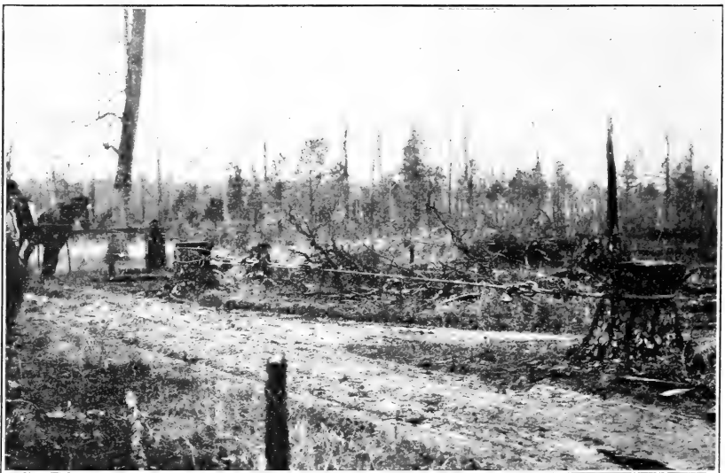
FIG. 5.—Capstan stump puller. This type requires an anchor stump from which all stumps within a radius equal to the length of the pulling cable can be pulled.
